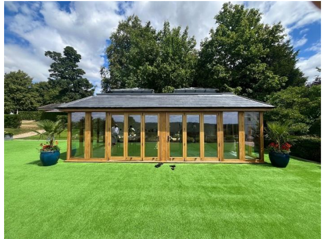
Photograph 2. The Garden Room building viewed from the west.
