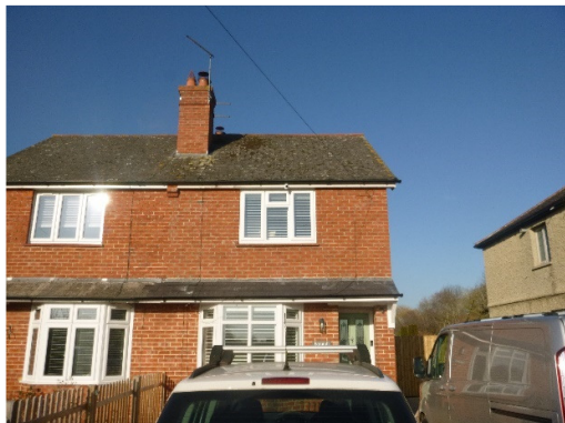
1. Front of the property viewed from the south
