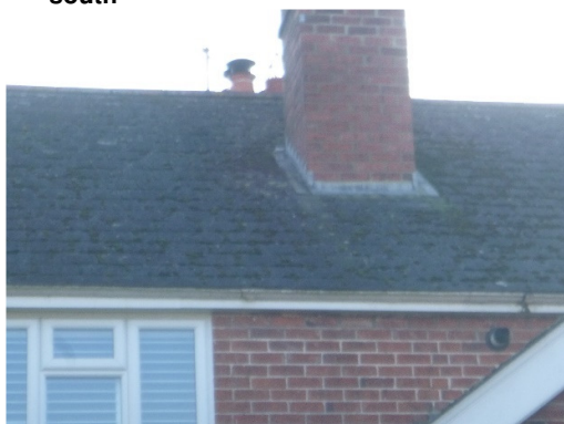
3. Tight slate roof tiles
