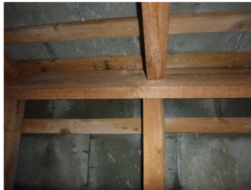
12. Asbestos lined tight slate roof tiles
