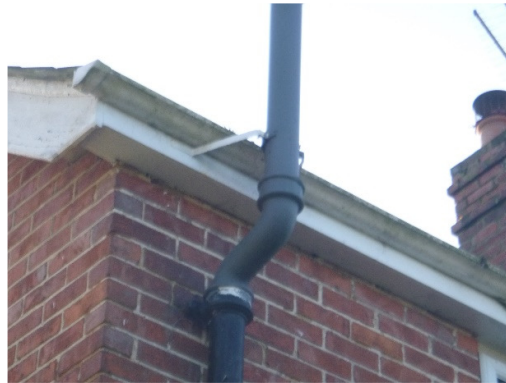
10. Soffits were tight to brickwork throughout
