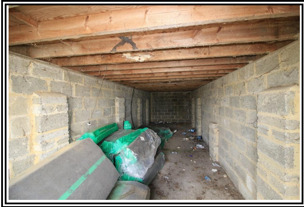
Photo 13: Building B Internal view central section
