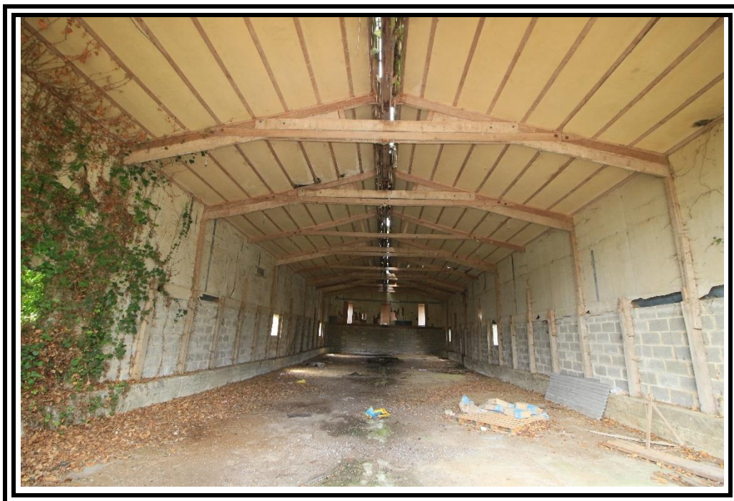
Photo 14: Building B: Internal view rear section
