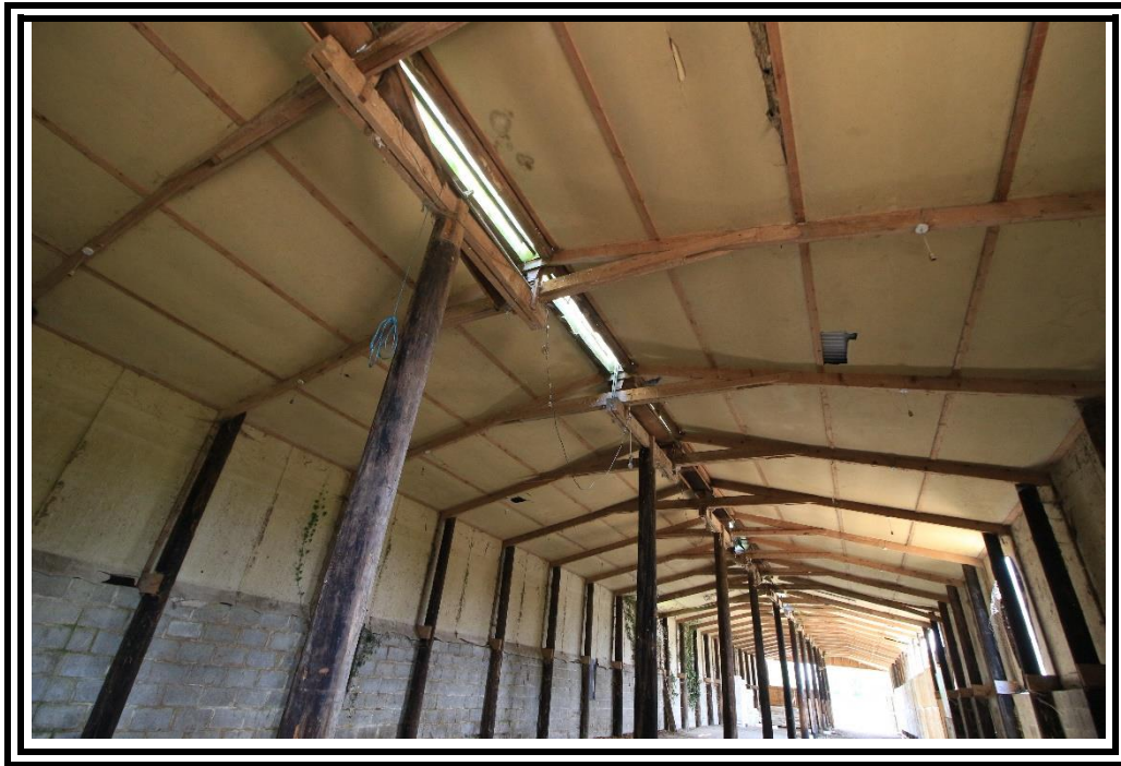
Photo 7: Building A : internal view
