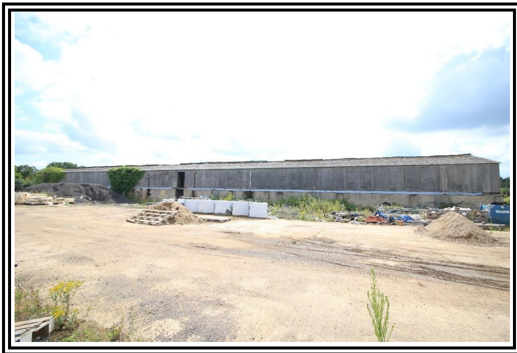
Photo 8: Building B: North side elevation
