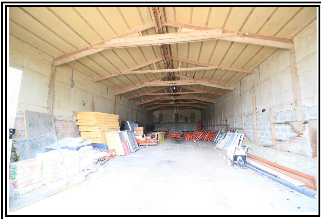
Photo 12: Building B Internal view front section
