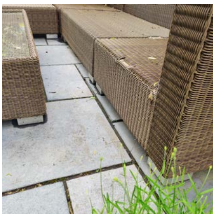
Distortion and lifting of the new patio.
