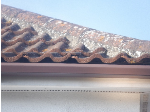
Photograph 5. Mesh present at the base of the roof tiles.
