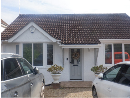
Photograph 1. Front of the bungalow viewed from the north.
