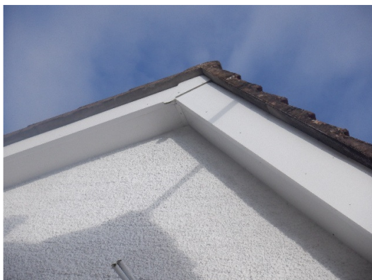
Photograph 8. Fascia tight to the rendered walls at the gable end to the western side of the bungalow
