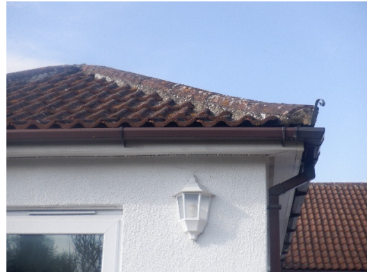
Photograph 4. Ridge and hip tiles mortared.
