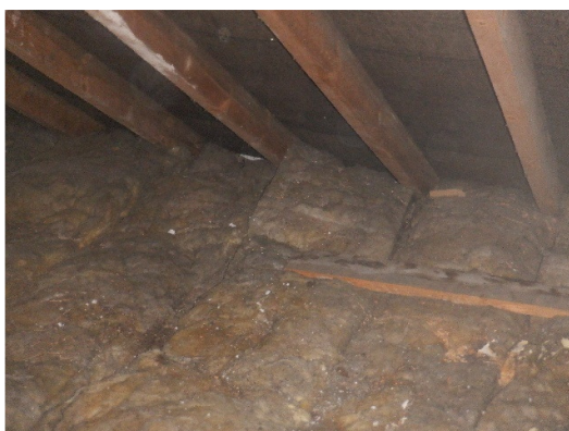
Photograph 13. Eaves filled to the front of the bungalow.
