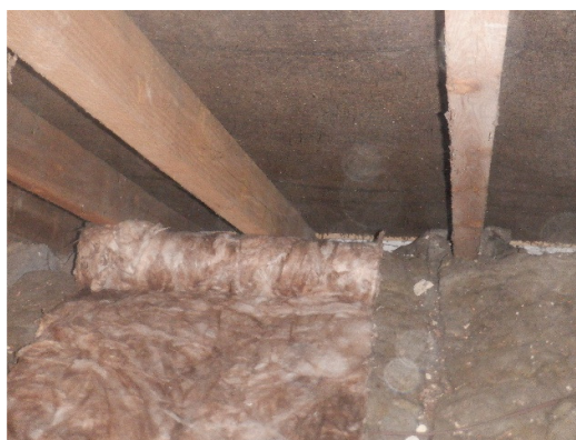
Photograph 14. Eaves open to the rear of the bungalow.
