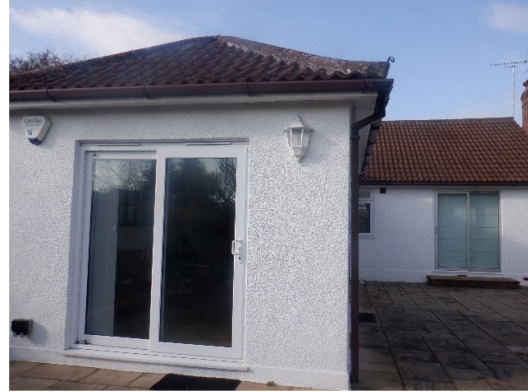
Photograph 2. Rear of the bungalow viewed from the south.
