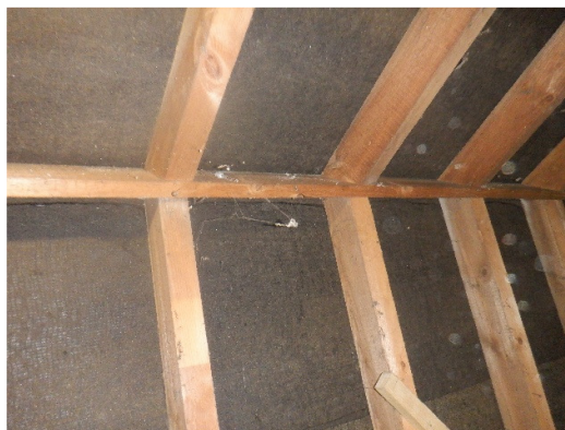
Photograph 11. Intact roofing felt..
