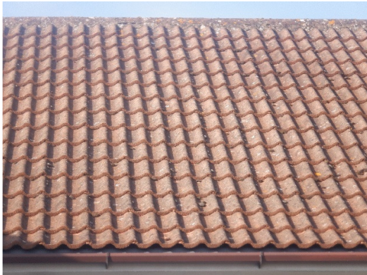
Photograph 3. Interlocking and intact roof tiles.
