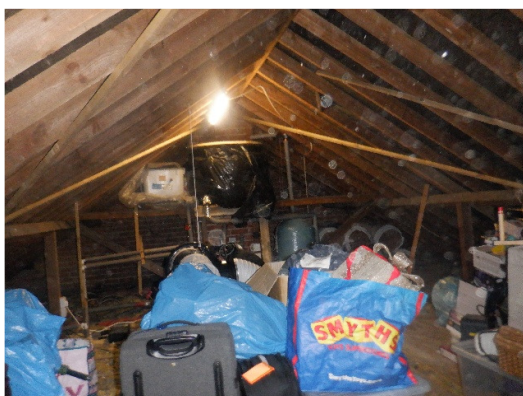
Photograph 10. Internal view of the roof void.
