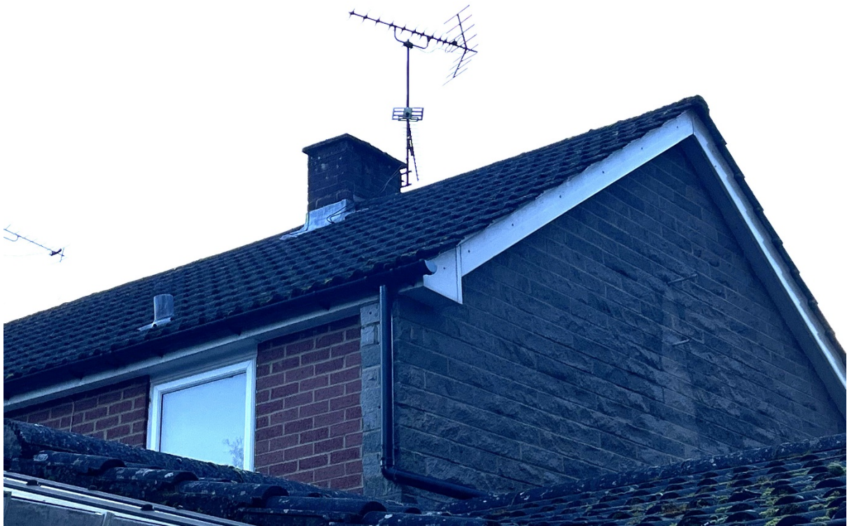
Figure 4. North gable looking southwest.
