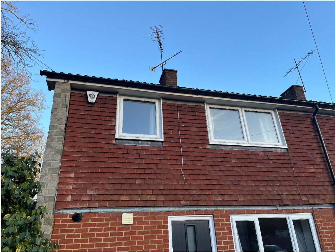
Figure 2. Western elevations looking east.
