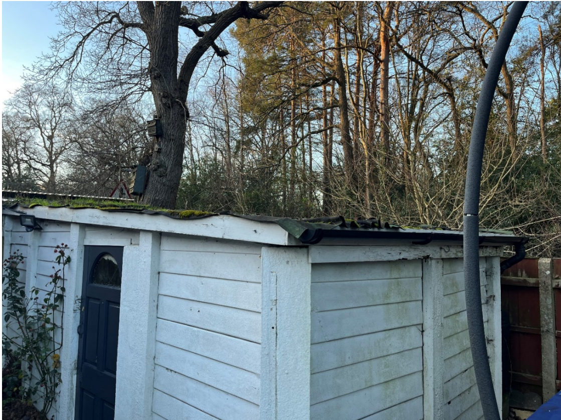
Figure 10. Garage looking northwest.
