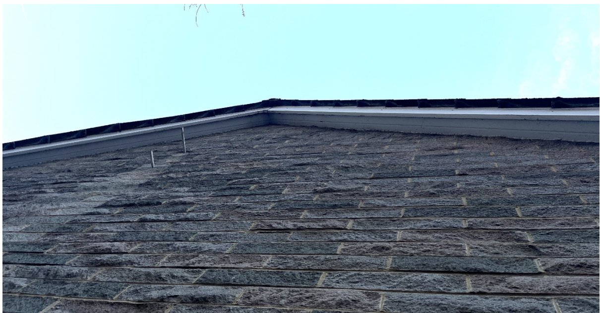
Figure 5. North gable soffits looking south.
