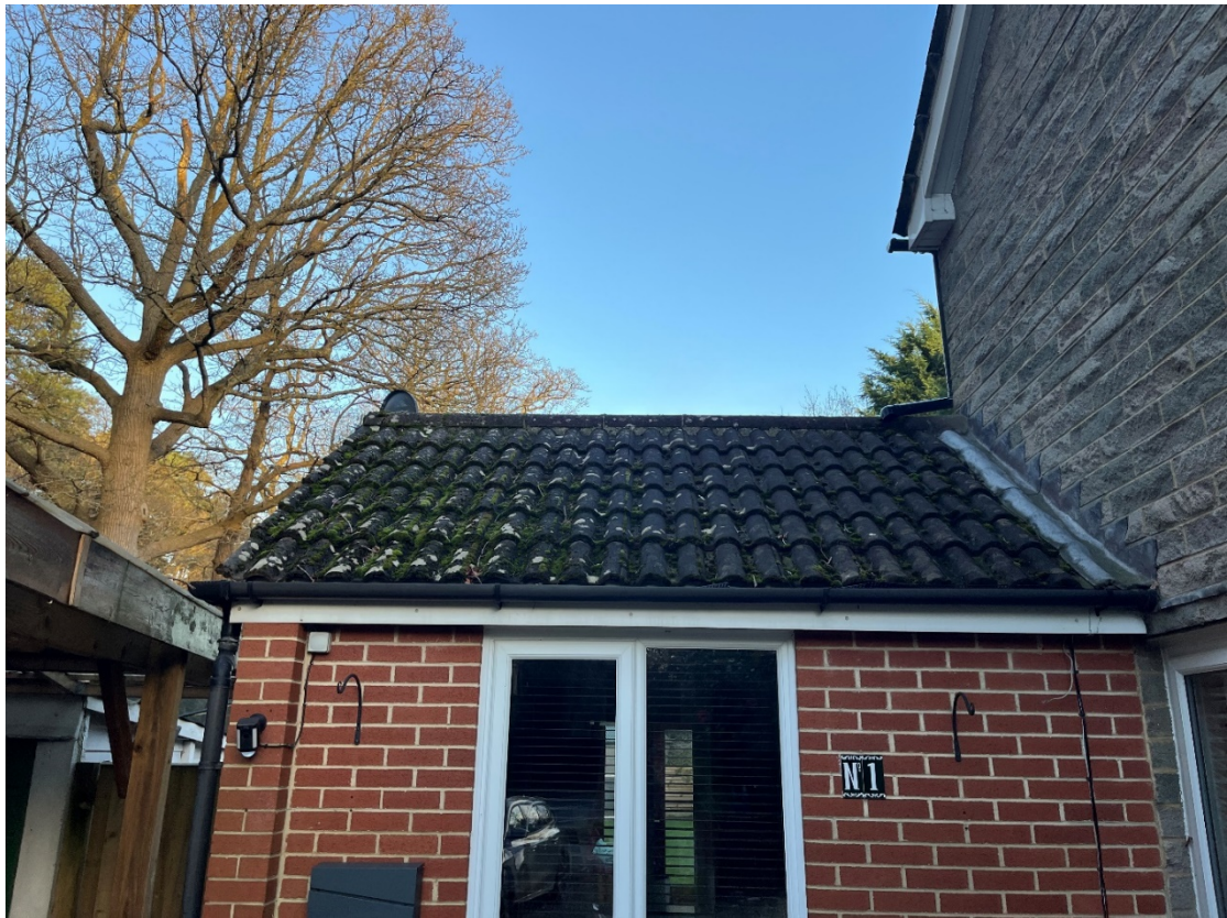
Figure 8. North ground floor extension looking east.
