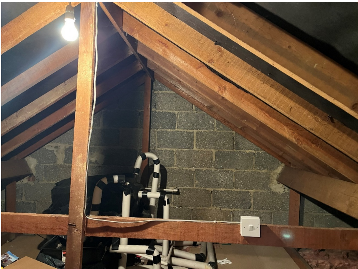
Figure 7. Loft looking south.
