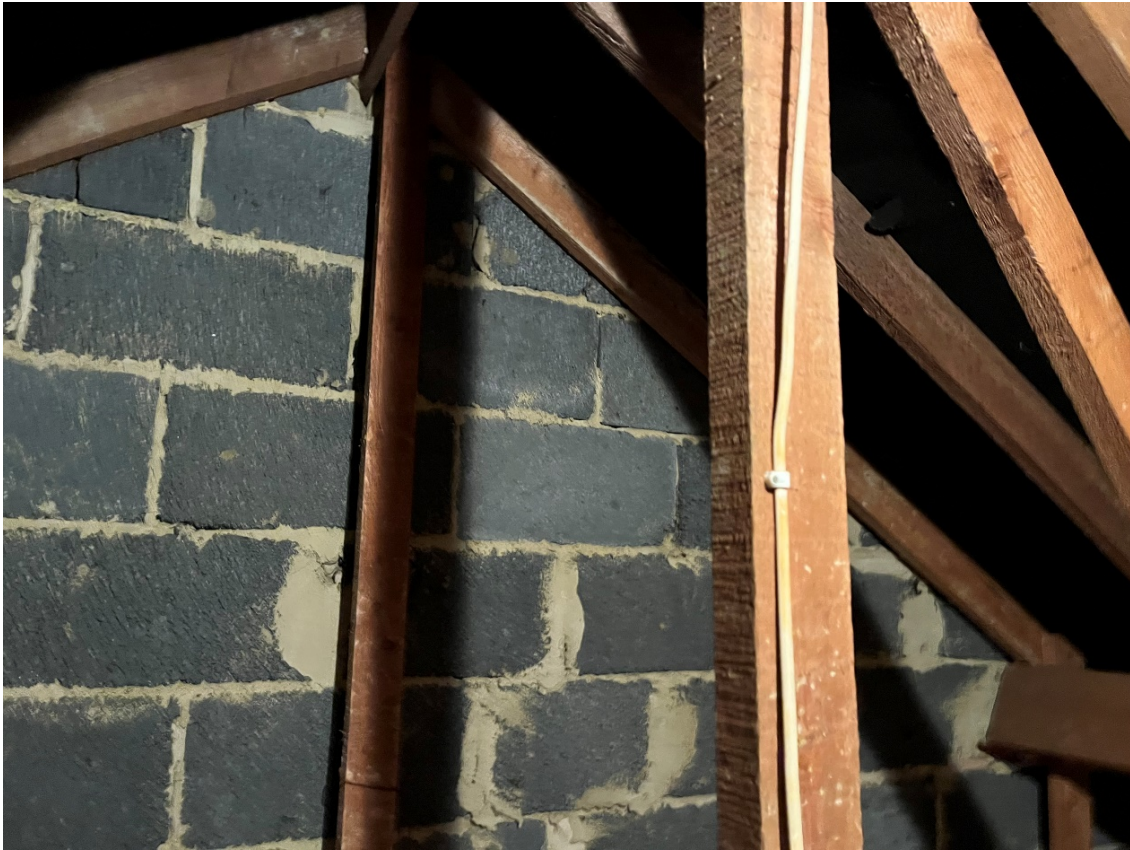
Figure 6. Loft north gable looking northeast.
