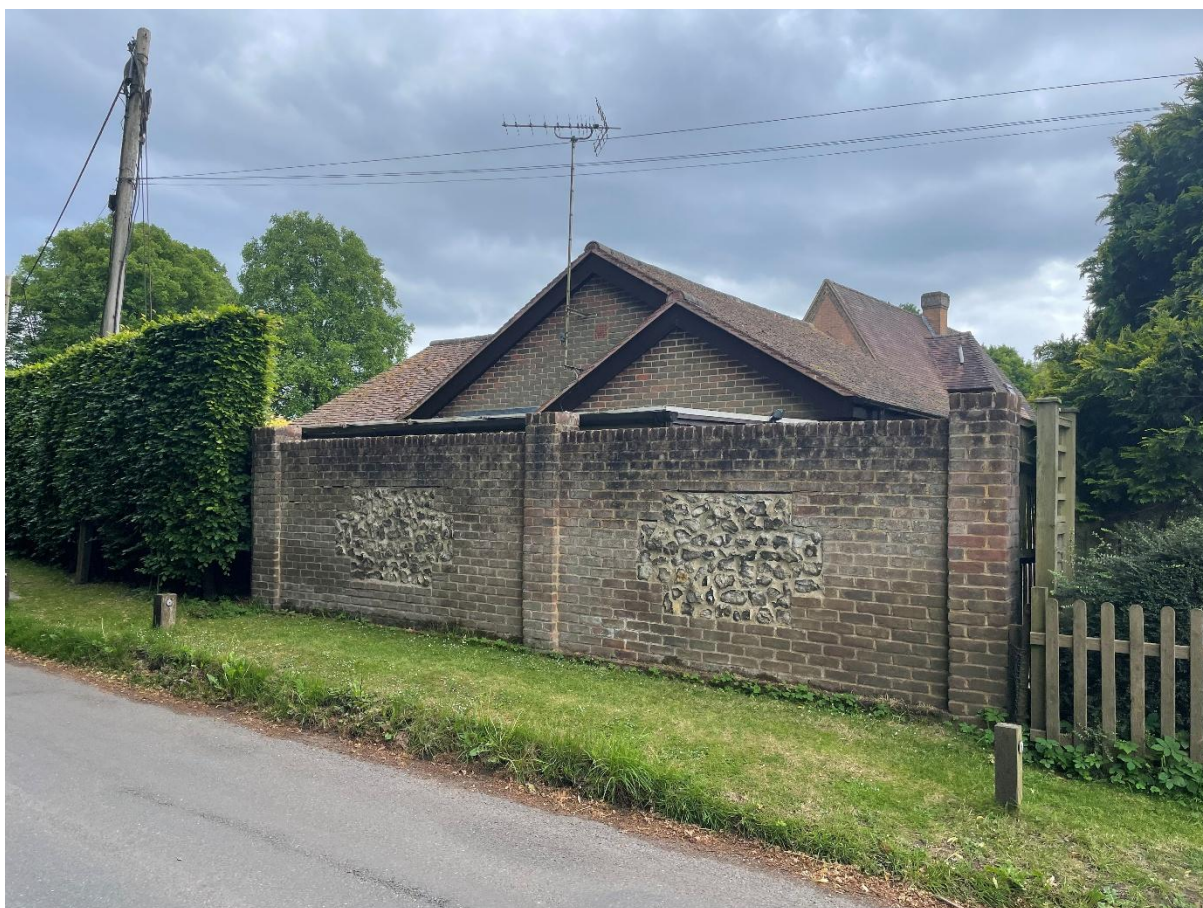
Photo 3: Example of wall, hedging and wide verges within the Area of Special Character, along Culham Lane.
