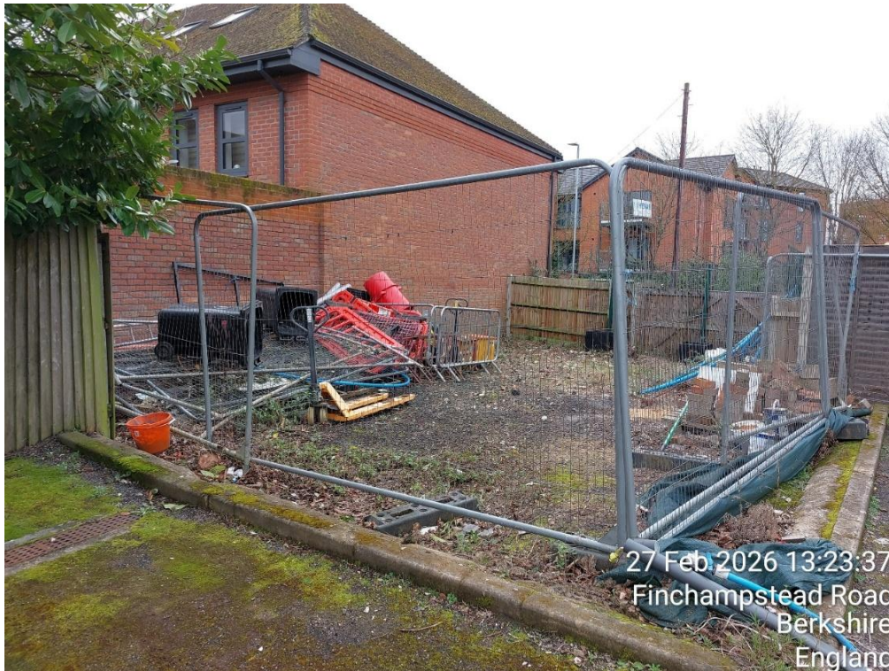
Photograph 01: view of site from the northeast
