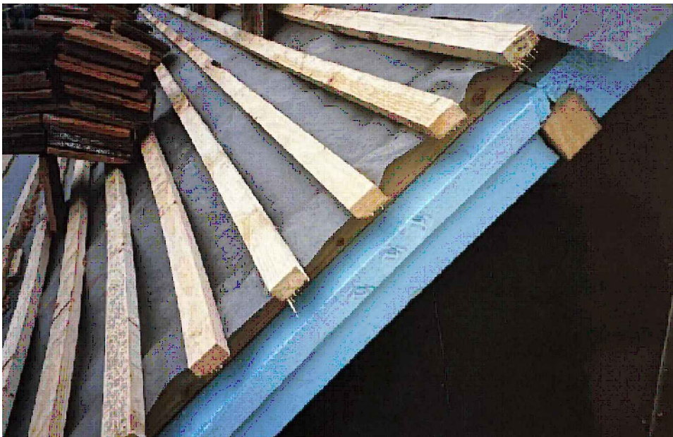
HISTORIC PHOTO TAKEN OF ROOF WHEN BEING PREVIOUSLY RETILED
