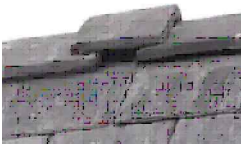
'Lifted' ridge tile (RT)
