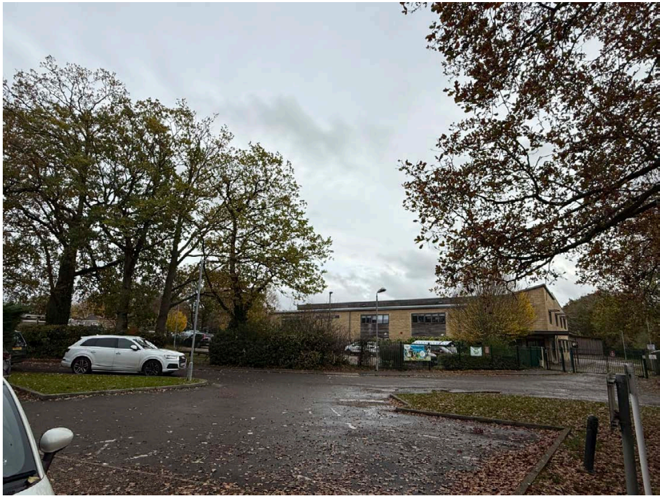
Parking area looking towards main entrance
