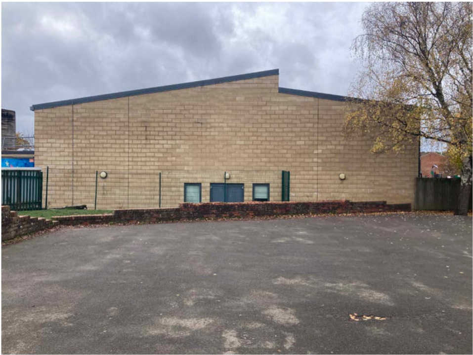
North East Elevation of existing Hall
