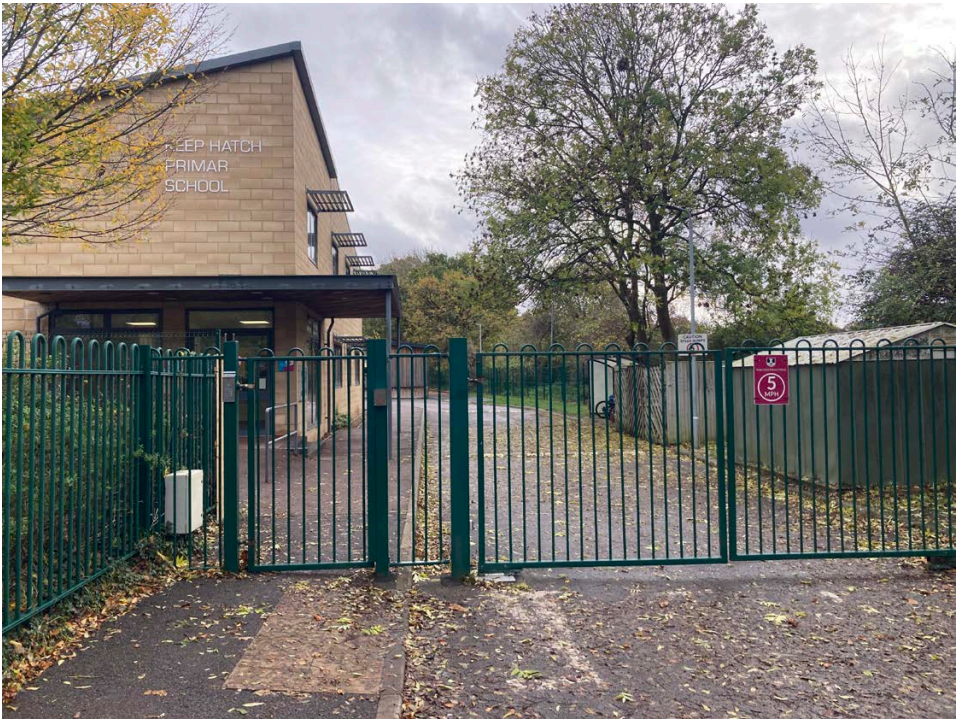
Main entrance gates
