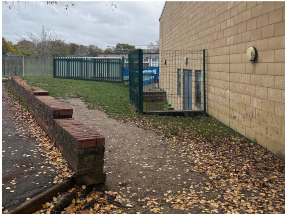
Changes in level at North East Elevation of existing Hall
