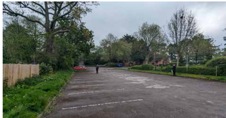
10. Existing parking area
