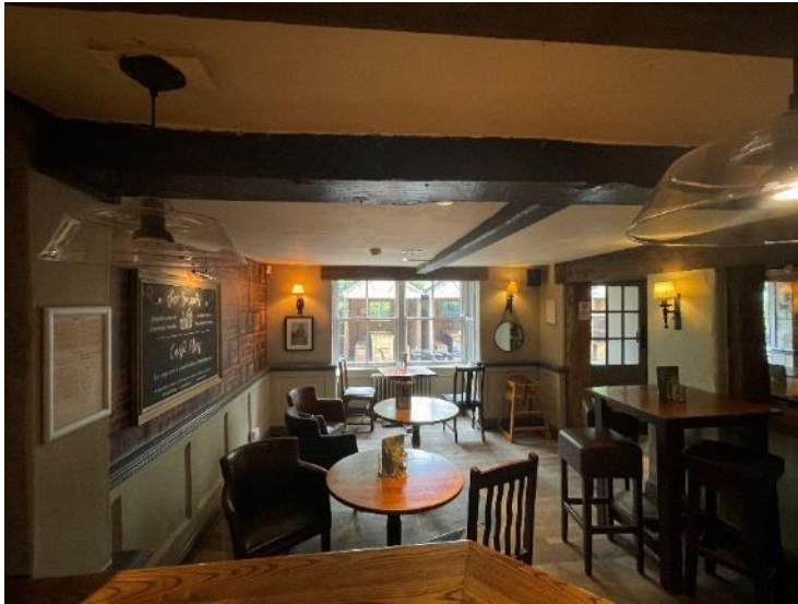
Plate 20: Front bar area, featuring ceiling timbers above.
