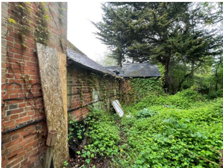
Plate 17: Eastern elevation fronting onto a small overgrown garden area.
