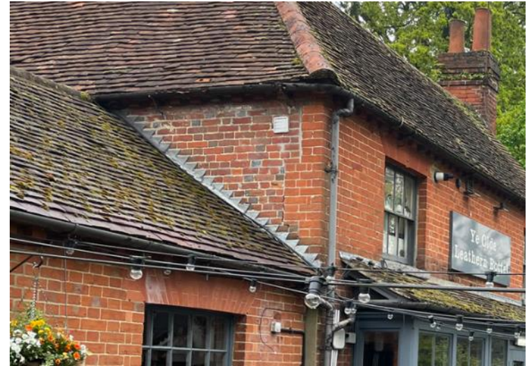
Plate 14: Evidence of alternative brickwork between the front and western side elevations.
