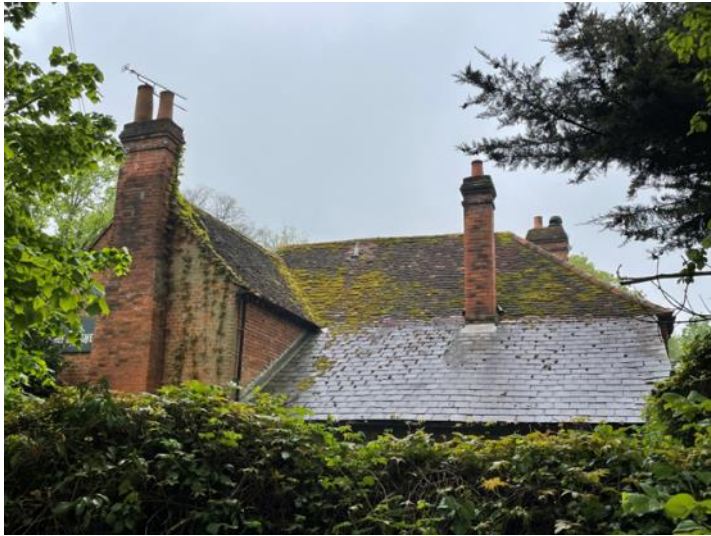
Plate 16: Main building roof, predominantly clay-tiled with small section of later slate tile.
