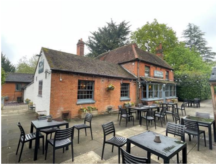
Plate 12: Front (south) Elevation.
