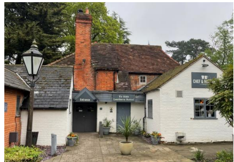
Plate 15: Western elevation, including modern additions at the ground floor and earlier building fabric above, including window.
