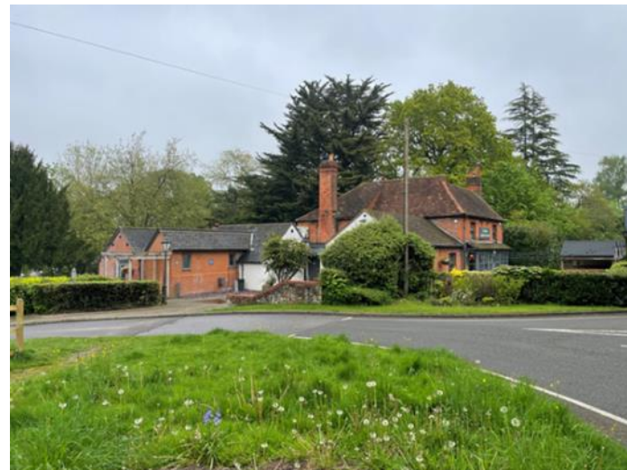
Plate 3: The wider extent of the Public House as seen from the southwest.
