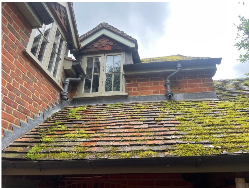
Plate 18: An image showing the roof on the lower level with multiple loose tiles which could provide entry points
