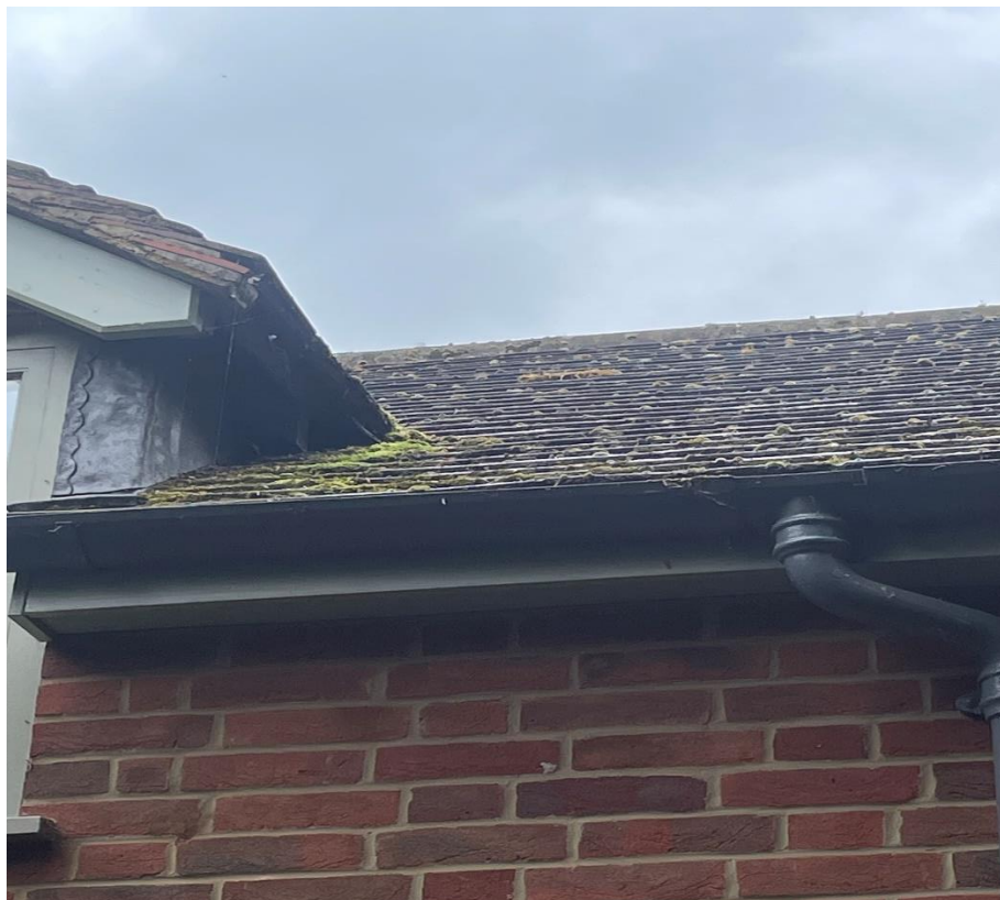
Plate 14: An image showing loose tiles on the roof and gaps in the soffit
