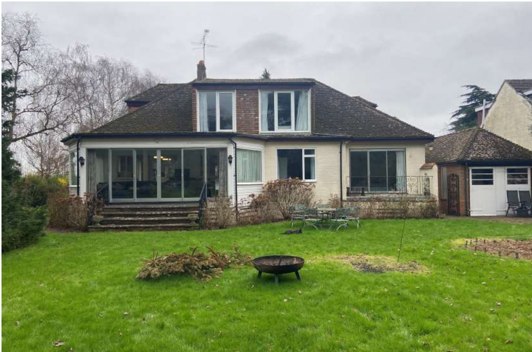
Figure 3: Existing rear elevation.
