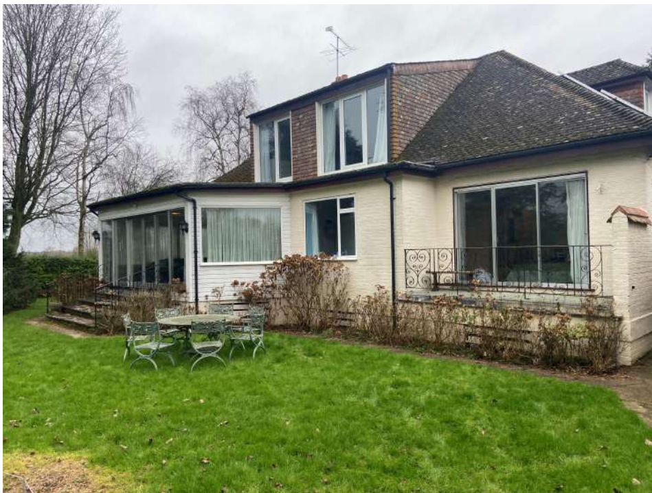
View of rear of house.
