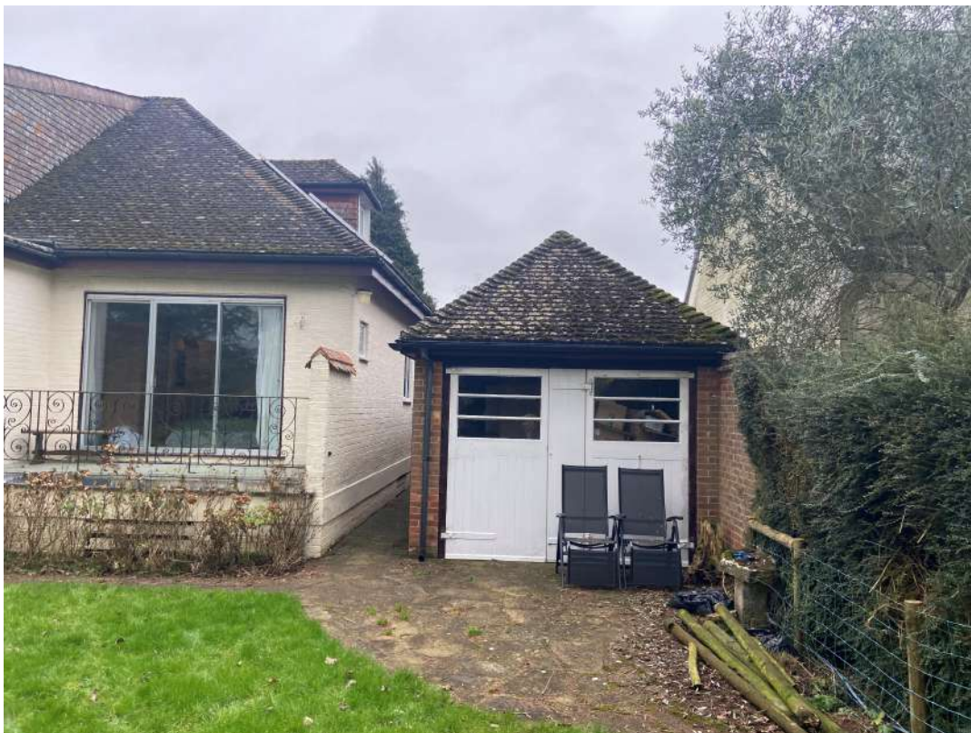
View of rear of garage.
