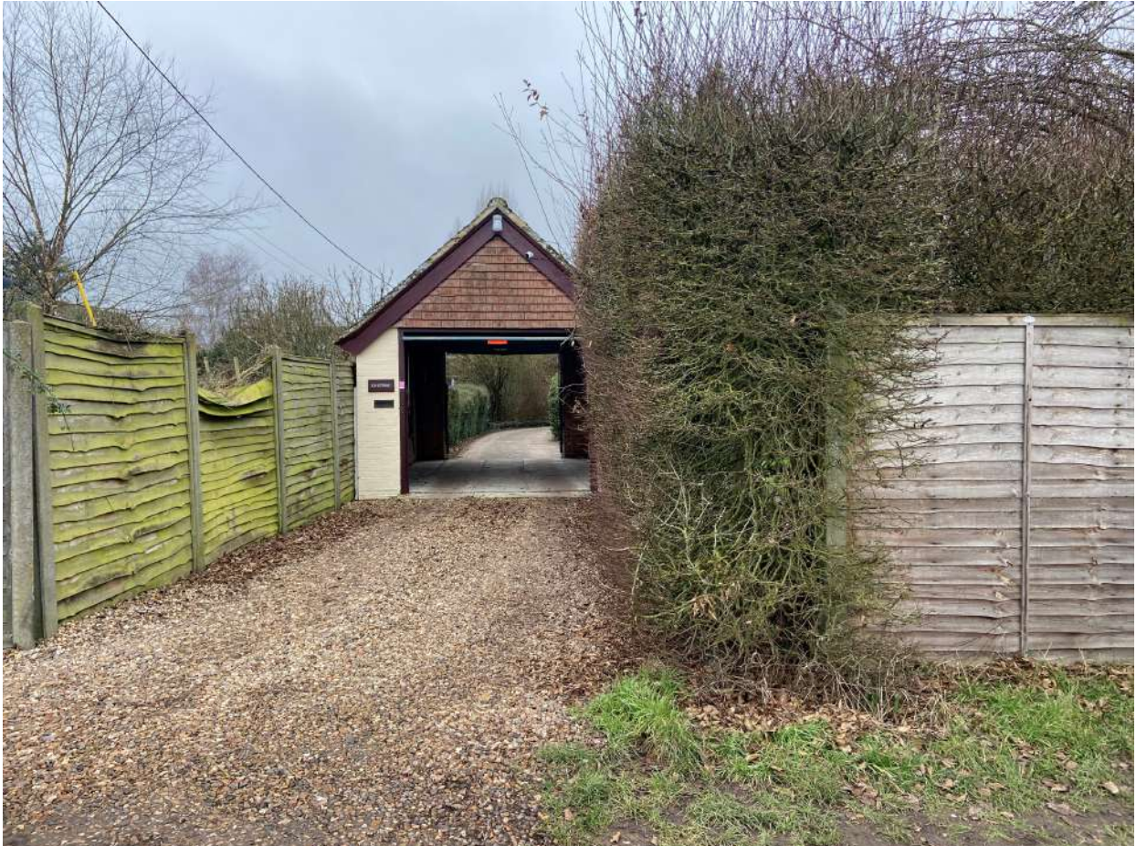
View of entrance to the site.
