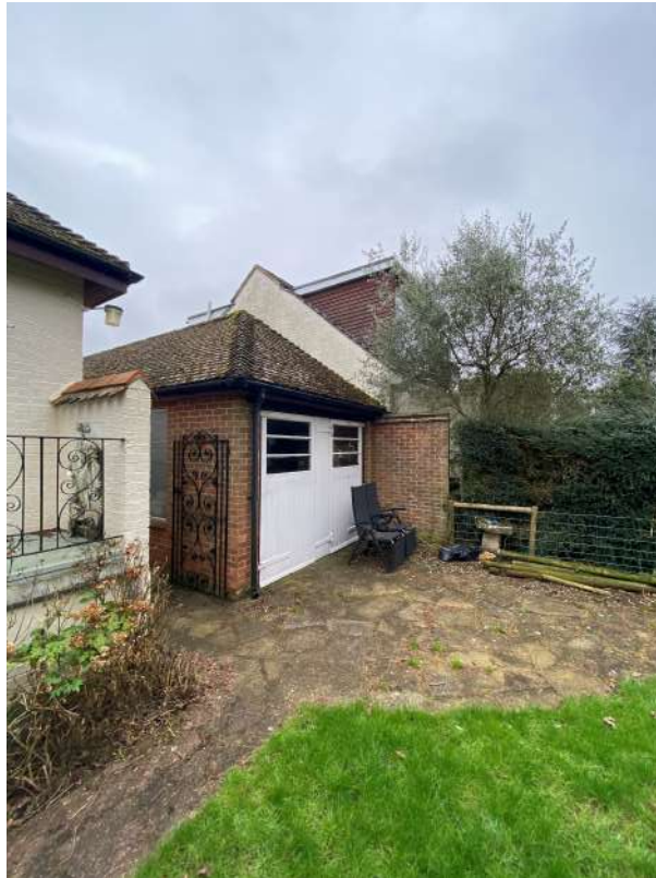
View of rear of garage.
