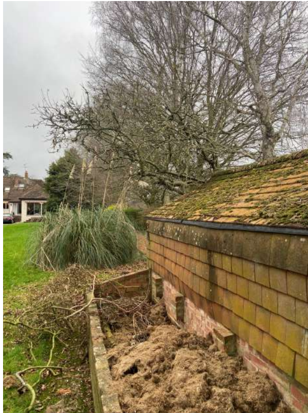
View along the north edge of site.
