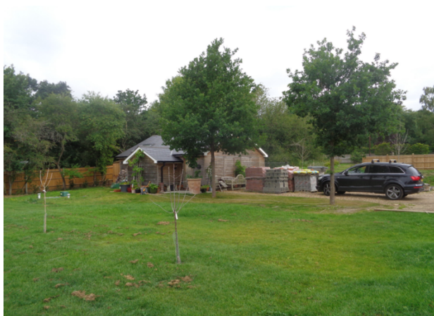
Figure 7 Moor Green Barn taken by Enforcement Officer on 14th July 2020
