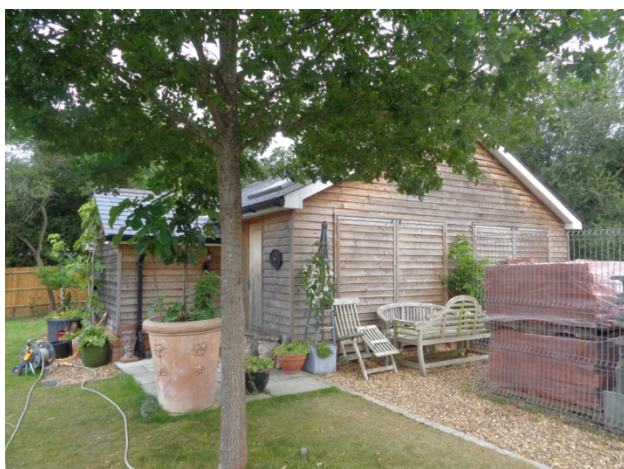
Figure 6 Moor Green Barn taken by Enforcement Officer on 14th July 2020
