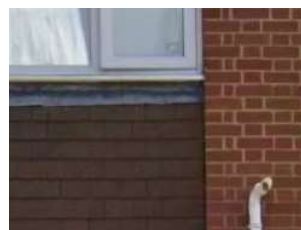
Red / Brown Clay Tiles on Facade
