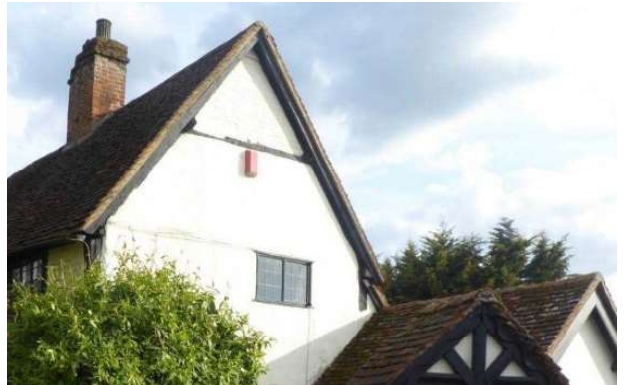
Figure 11. Gable Roof (Rightmove)
