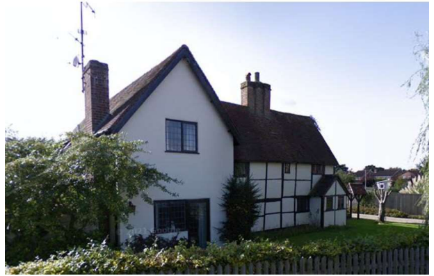
Figure 10. Front elevation to White Cottage (Google Street View, 2008)
