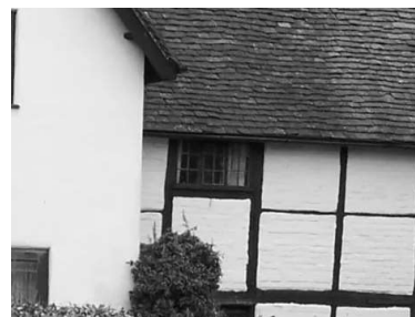
Original 16c Irregular Black Timber Leded Casement Windows
