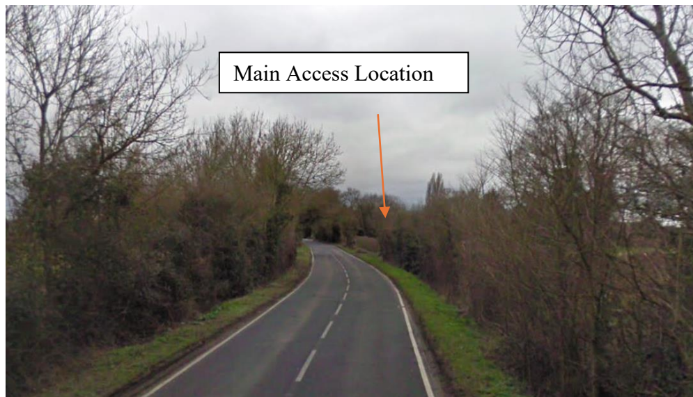
Fig 12. Google Street View showing the location of Access Road onto Lodge Road (north)
