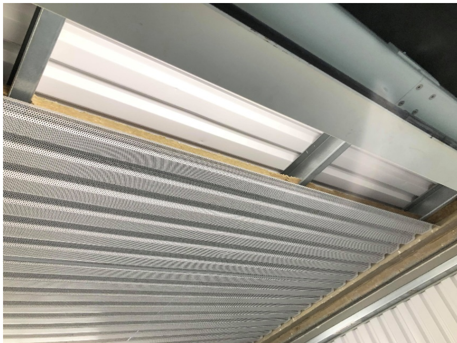
Image 1 - Enhanced Acoustic Specification inc. Underdrawn Perforated Liner
