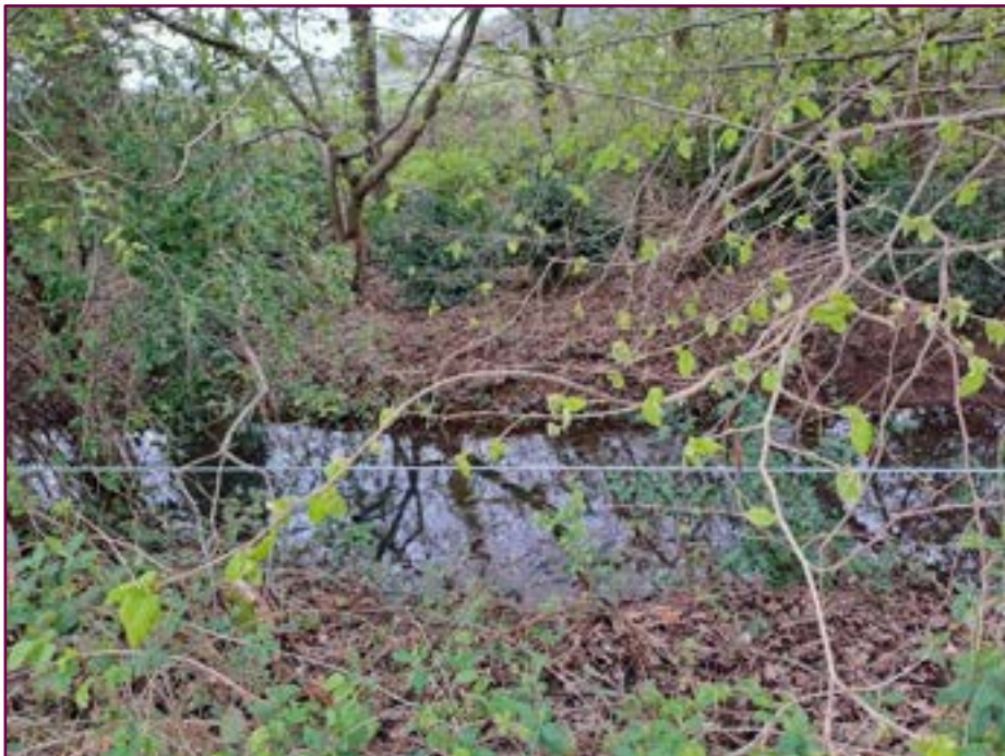
Figure 3. Drainage ditch on southern boundary
