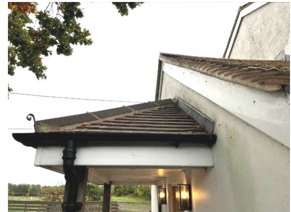
Photograph 6. Flush lead flashing Intact hip mortar on porch roof and intact verge mortar (northern elevation).
