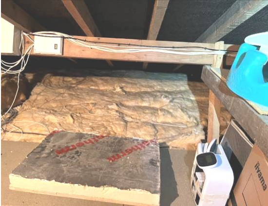
Photograph 13. Fibreglass insulation along sides and blocking eaves (roof void).
