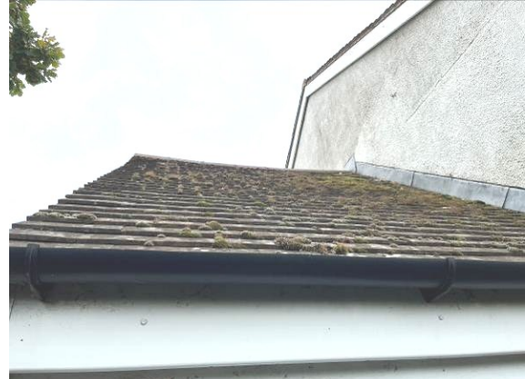
Photograph 4. Flat overlapping roof tiles (western elevation).
