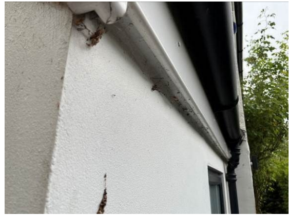
Photograph 8. Soffit tight to wall (western elevation).
