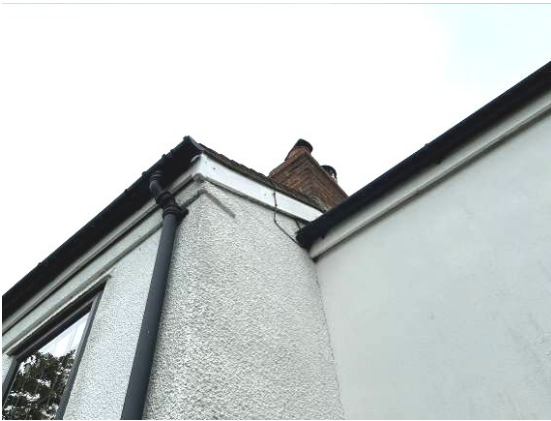
Photograph 7. Tight barge board to gable and wall (eastern elevation).
