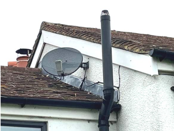
Photograph 5. Intact verge mortar and flush lead flashing and fascias (southern elevation).
