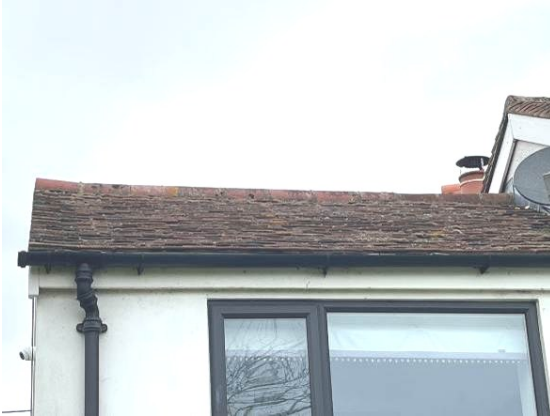
Photograph 3. Tight ridge tiles (eastern elevation) (proposed location of extension).
