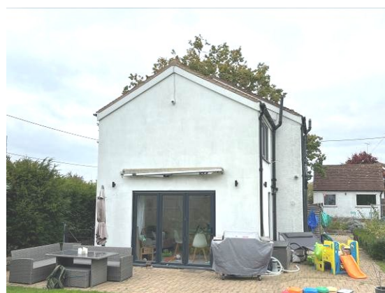
Photograph 2. Rear of the property viewed from the south.
