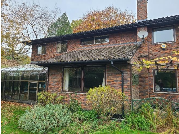
Photo 3 – external view of building 1 interlocking roof tiles.
