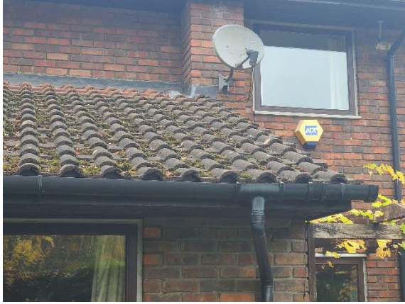
Photo 3 – external view of building 1 interlocking roof tiles.
