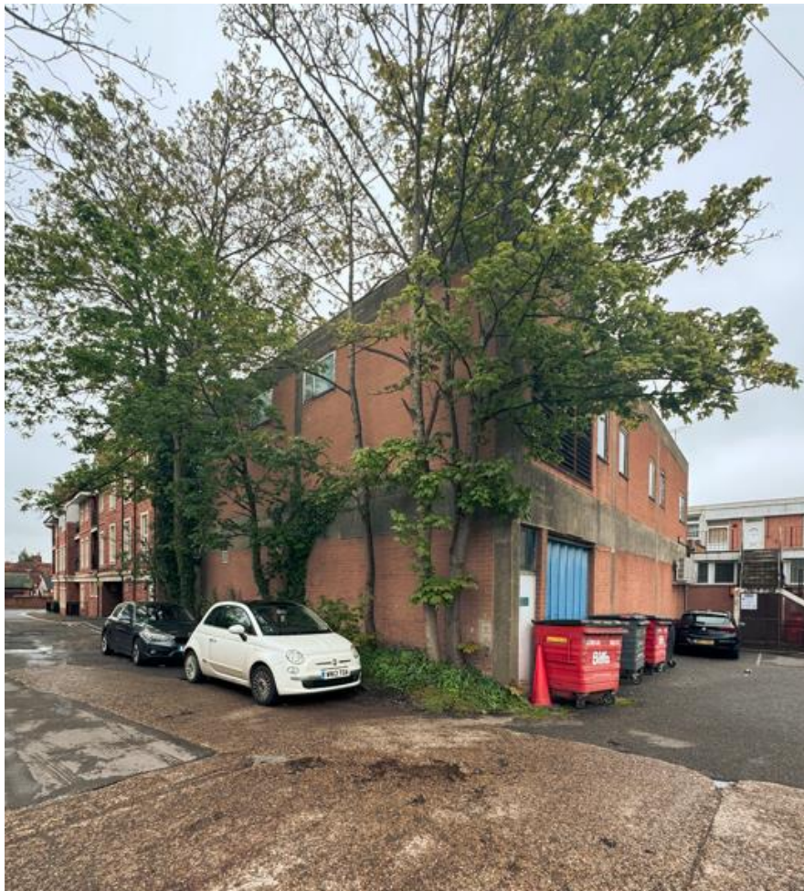
Pl.2: The building to the rear of Nos.68-70 Peach Street from the north-west.
