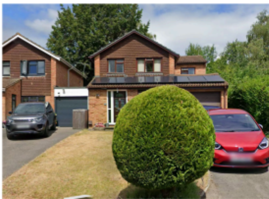
Google Street View image from street level
