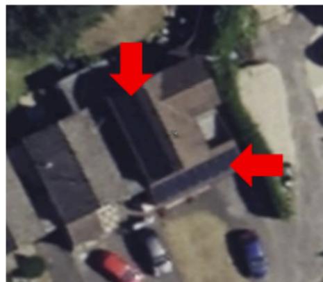
Bing aerial photograph of the roof configuration
