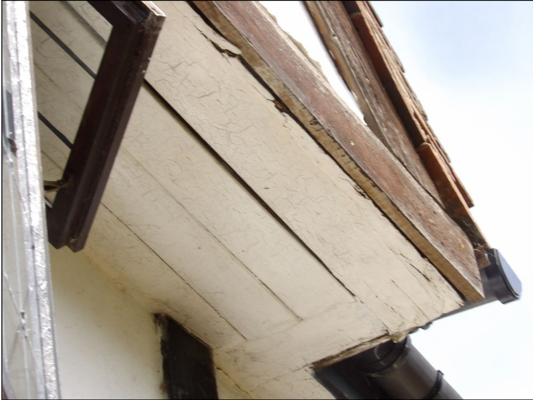
Figure 9. Gaps in soffits of overhang over bay window. 6 Old Bath Road, Sonning. 20.05.25
