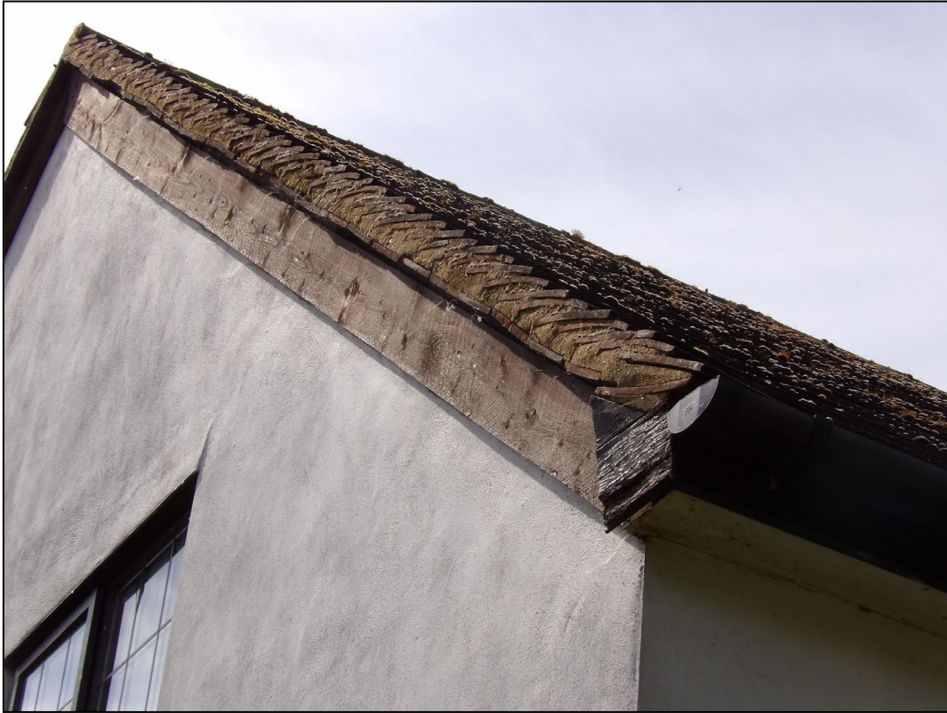
Figure 7. Example sealed verges. 6 Old Bath Road, Sonning. 20.05.25
