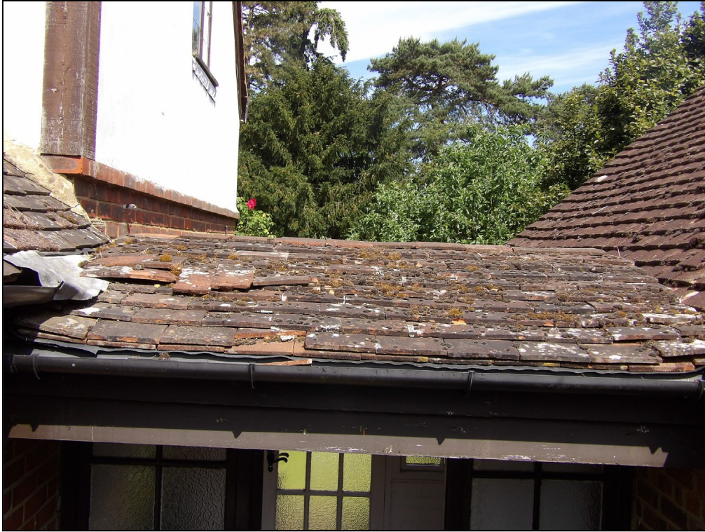
Figure 11. Raised tiles on link building. 6 Old Bath Road, Sonning. 20.05.25
