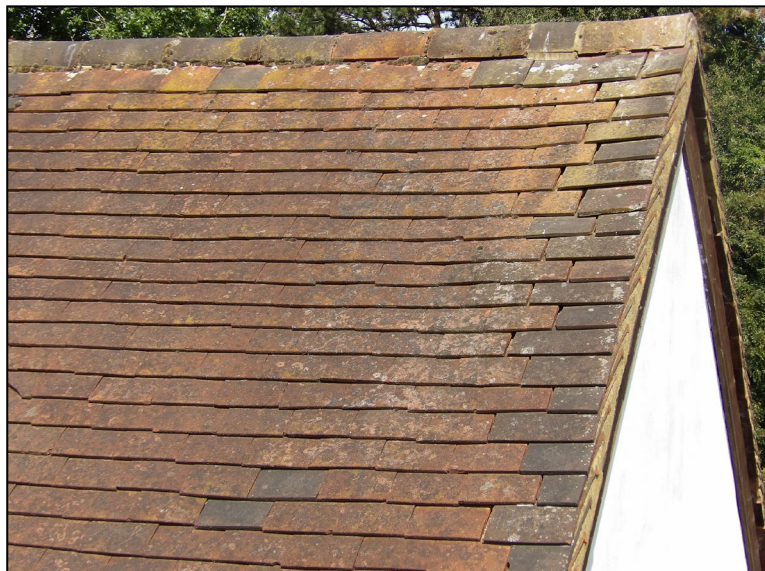
Figure 6. Example missing mortar from ridge tiles and moved tiles. 6 Old Bath Road, Sonning. 20.05.25
