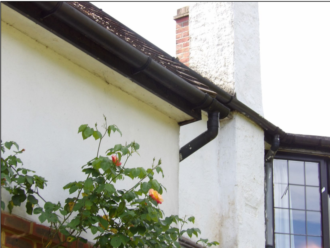
Figure 8. Example sealed soffits/fascias. 6 Old Bath Road, Sonning. 20.05.25
