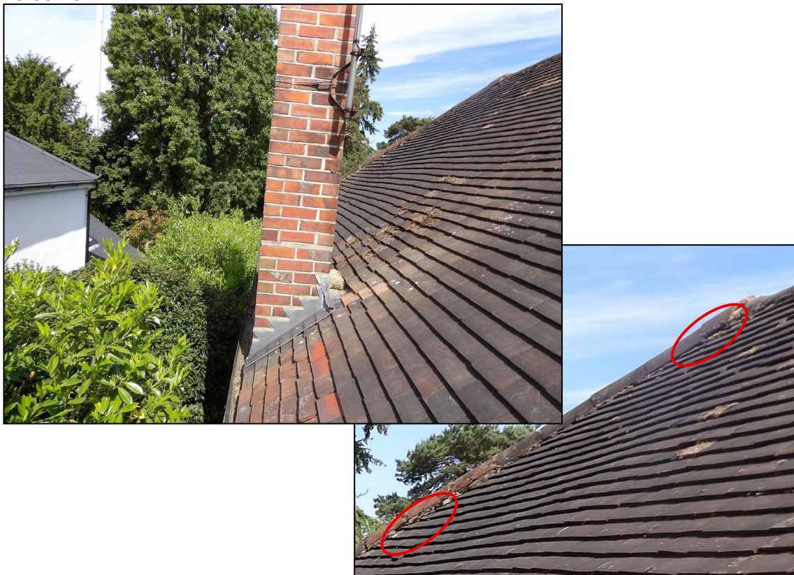
Figure 6. Example missing mortar from ridge tiles and moved tiles. 6 Old Bath Road, Sonning. 20.05.25
