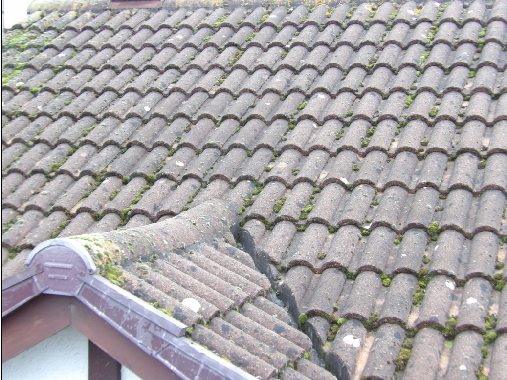
Figure 5. Sealed roof/ridge tiles, valleys and verges on dormer on front elevation. 22 Beaver Way, Woodley. 17.12.24
