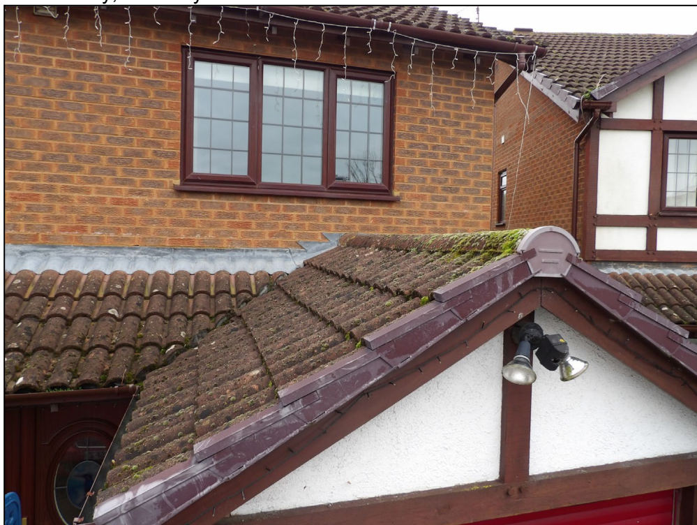
Figure 8. Example sealed roof and ridge tiles and verges on part attached garage. 22 Beaver Way, Woodley. 17.12.24
