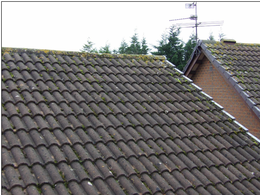
Figure 4. Example of roof/ridge tiles and verge clips. 22 Beaver Way, Woodley. 17.12.24
