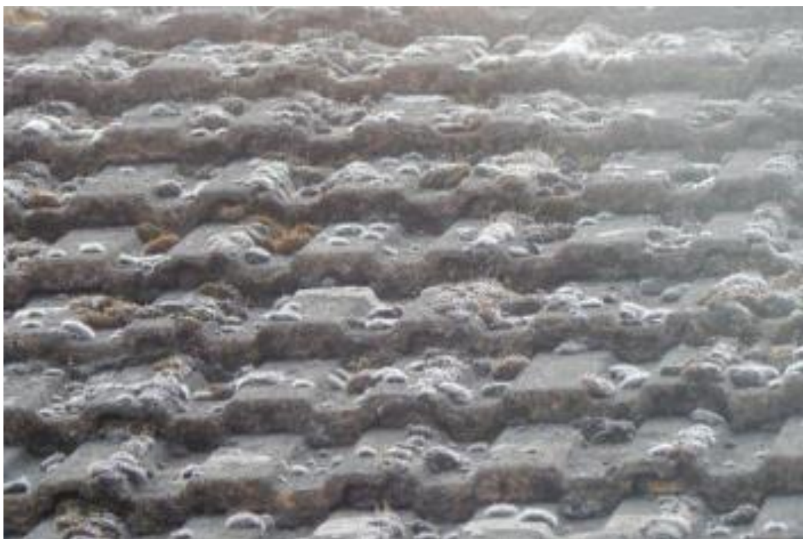
Image 5 – Close view of the rear roof coverings
