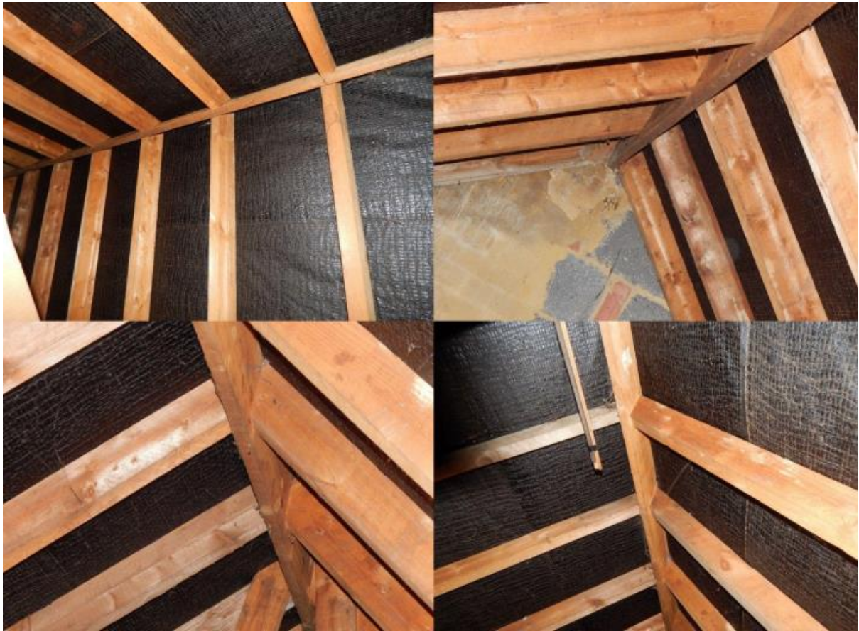
Image 9 – Internal view from within the main roof void spaces
