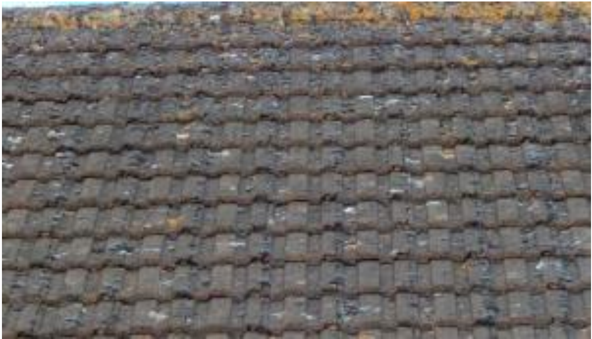
Image 3 – Close view of the front East facing roof coverings
