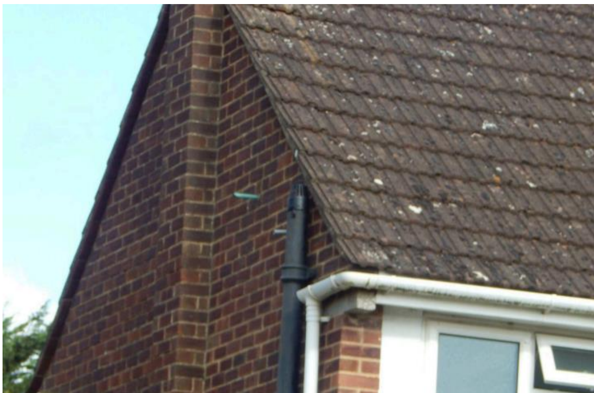
Image 6 – South facing elevation of the property
