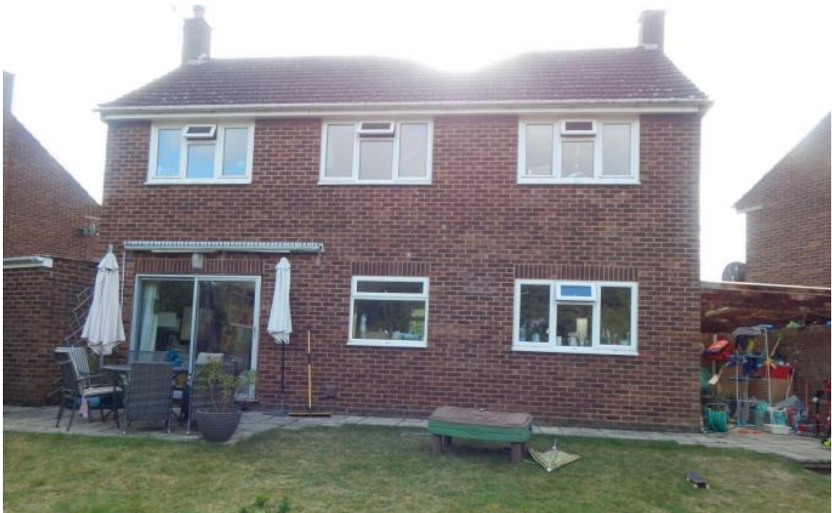
Image 4 – Rear West facing elevation of the property
