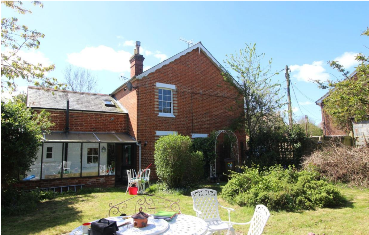
Rear and northern side of No. 27, showing the original two-storey gable and later low-level additions
