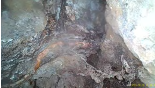
Photo 3: Ceiling of PRF 1
