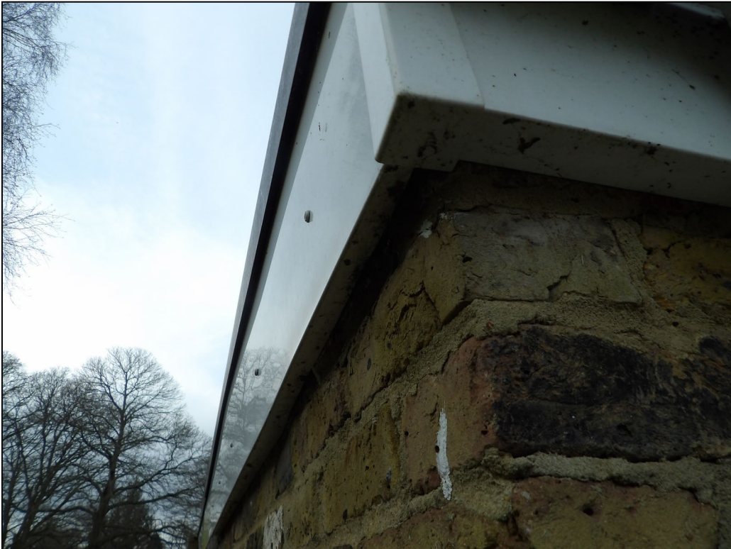
Figure 10. Sealed fascias on garage. 216b Nine Mile Ride, Wokingham. 21.01.25
