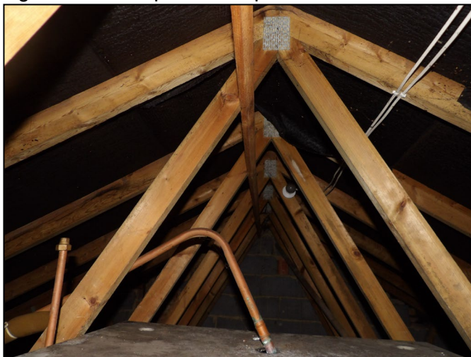
Figure 11. Example of loft space. 216b Nine Mile Ride, Wokingham. 21.01.25
