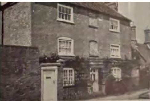
Fig 5.5 Historic photograph of side entrance with taller wall
