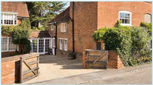
Fig 5.6 Recent photograph of solid timber vehicle entrance gate
