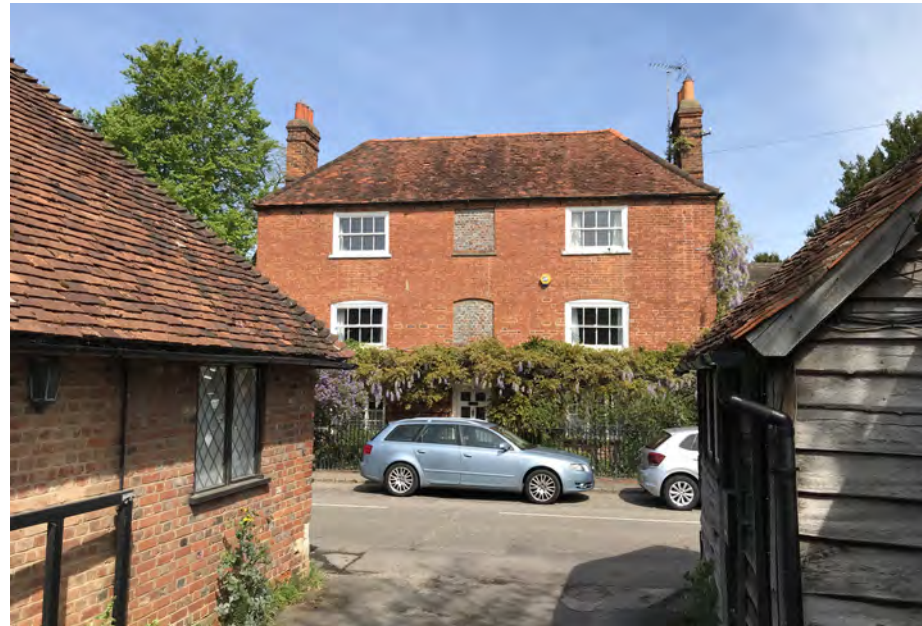
fig 2.6 View of Sonning House from car park behind the Old Forge.
