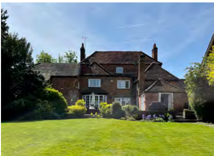
Fig 4.3 Existing rear photograph
