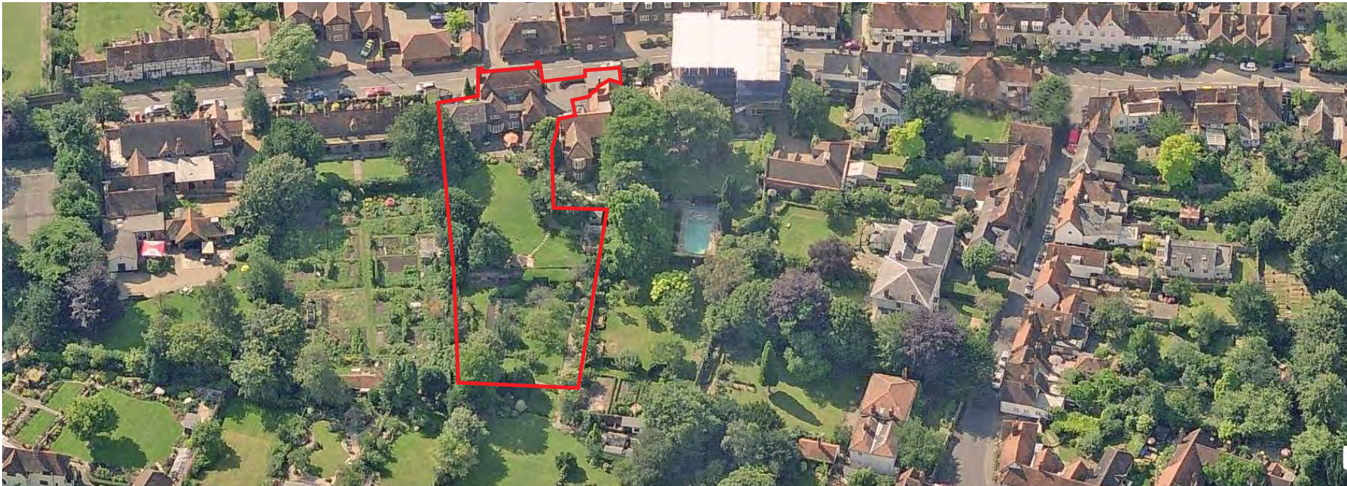
fig 2.5 View Looking South
