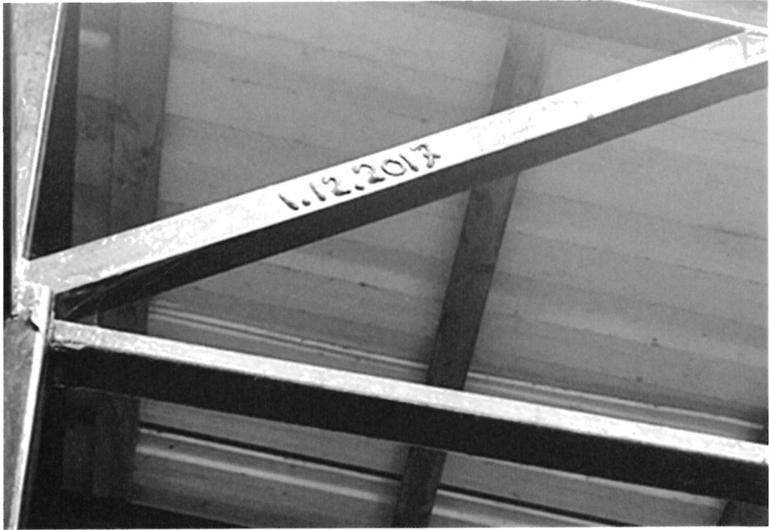
Internal beam in Building A
