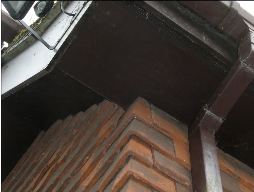
Figure 8. Front corner hanging tiles with gaps. Brook House, Hollybush Ride, Finchampstead. 05.12.23
