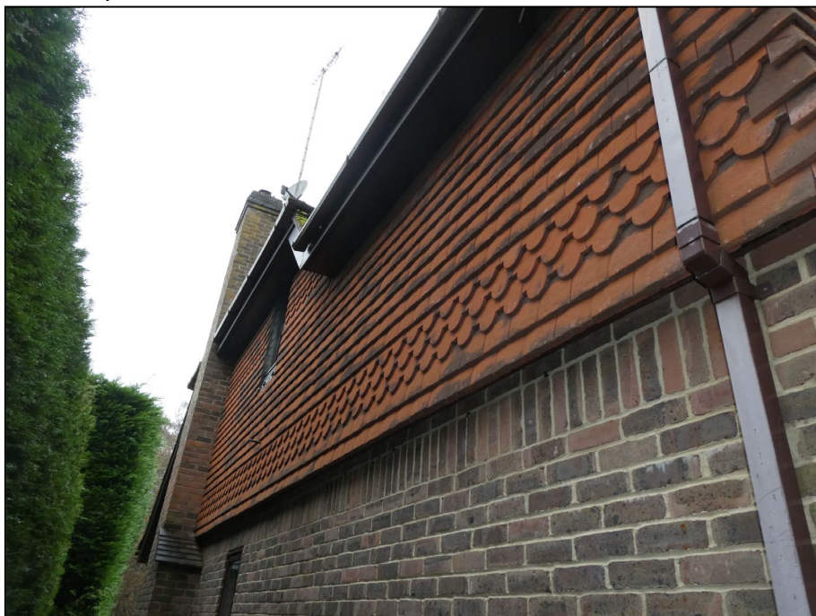
Figure 7. Example of tight-fitting hanging tiles. Brook House, Hollybush Ride, Finchampstead. 05.12.23
