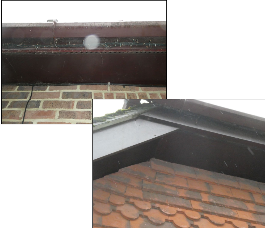
Figure 6. Example sealed soffits/fascias. Brook House, Hollybush Ride, Finchampstead. 05.12.23
