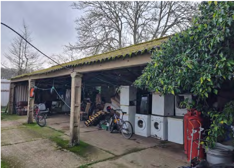
Photograph 2: Open-sided storage barn located on-Site, including some domestic white goods and objects, as well as two gas tanks, located in the east of the Site. Potential ACMs are present within the barn's building fabric.
