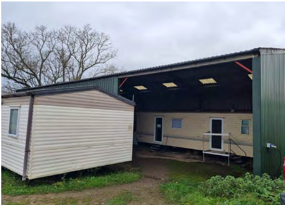
Photograph 4: One of the existing barns used for caravan storage, as well as a second caravan located adjacent to the barn, located in the east of the Site.
