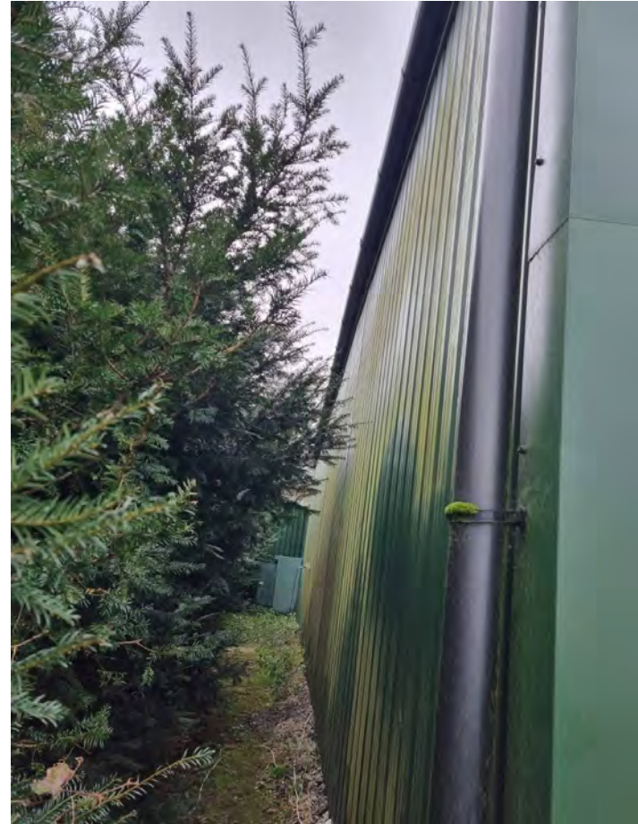
Photograph 10: Close up of the exterior construction of one of the existing barns.
