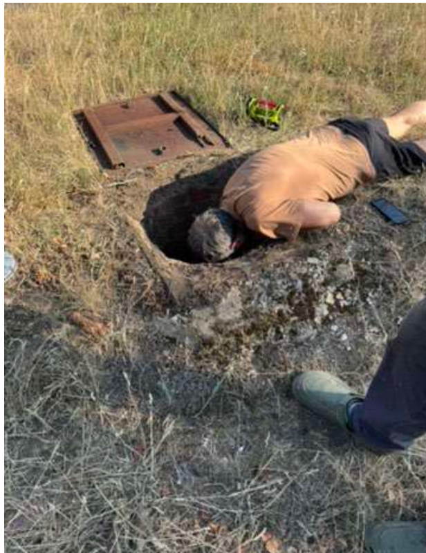
Hurst resident examining storm drain on Triangle.
