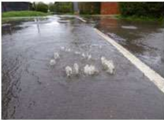
Hogmoor Lane manhole discharge going down Hogmoor Lane
