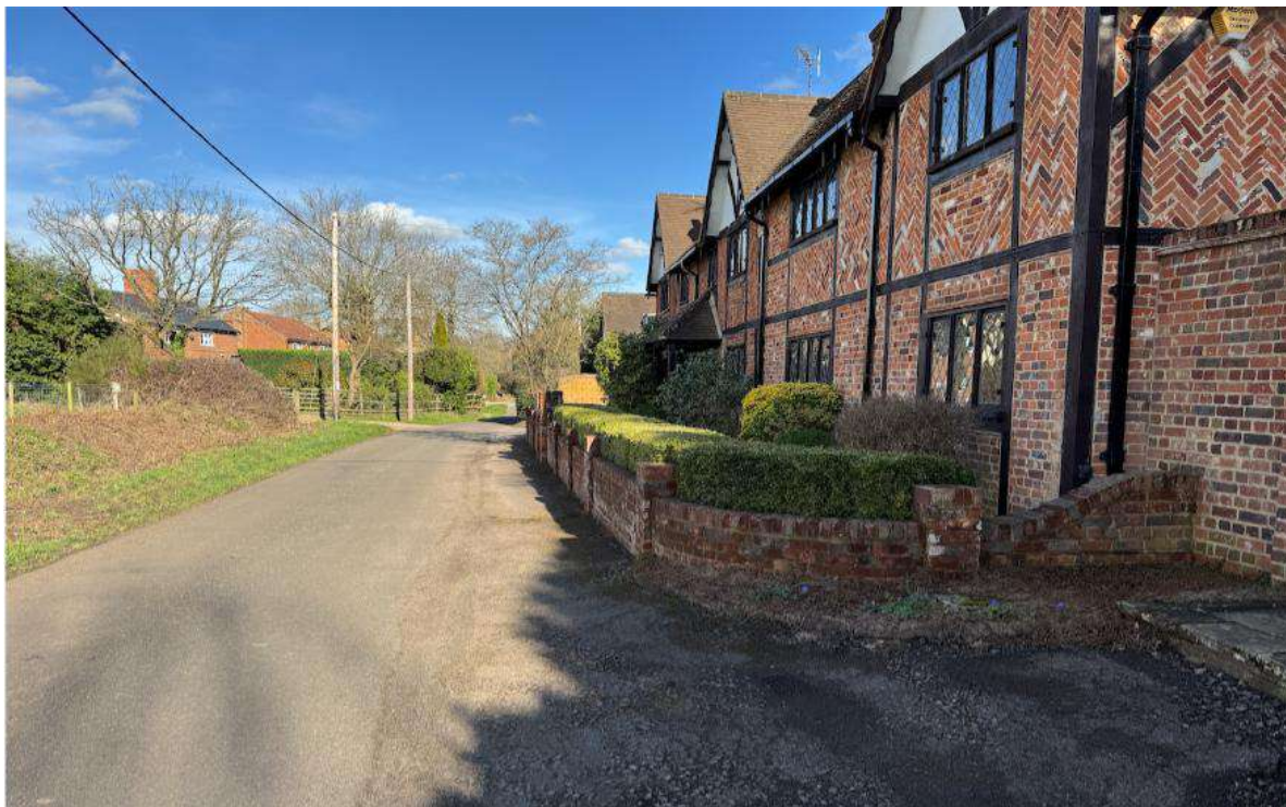
Fig. 12: View, looking north-east along Hogmoor Lane, with the frontage of Munfin House to the right.
