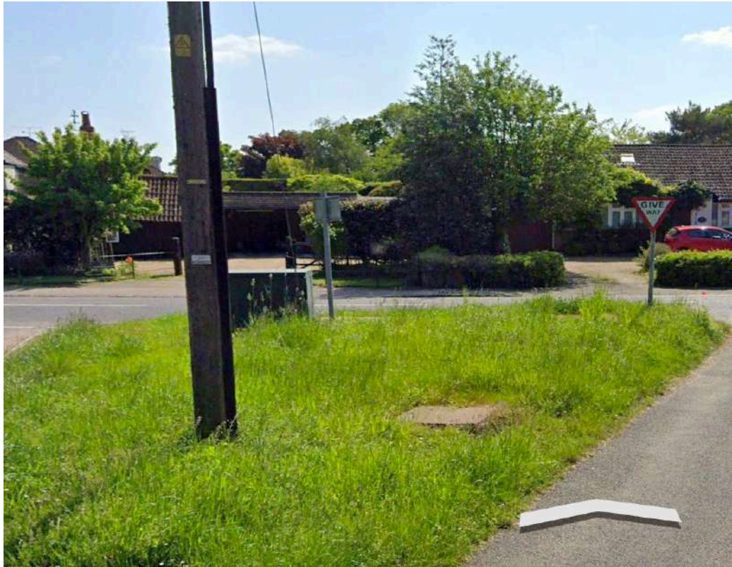
Grassy Triangle from R hand branch of Y junction showing manhole cover over 8 feet deep storm drain.
