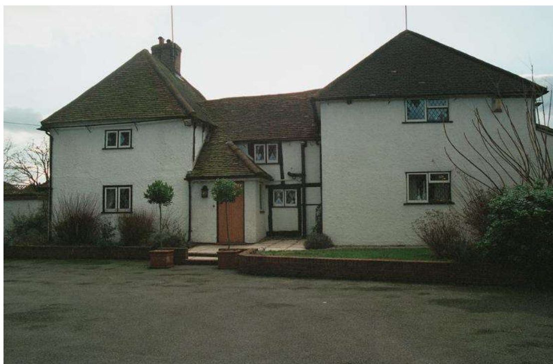
Fig. 10: View, looking south, of the rear elevation of Wards Cross House (Historic England).
