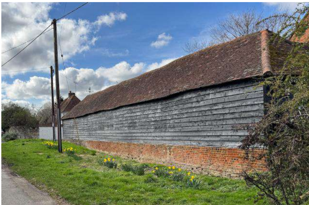
Fig. 13: View, looking west from Hogmoor Lane, of the road frontage of Long Barn.
