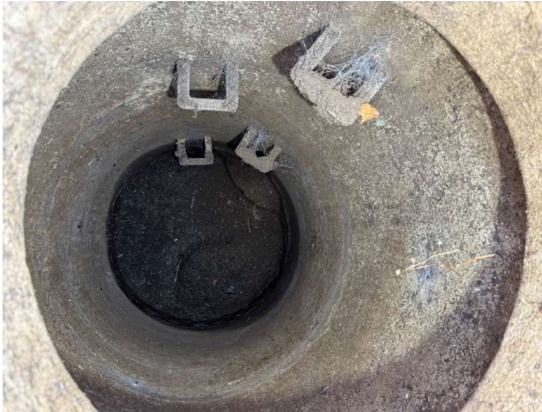
Close up of entrance to storm drain.
