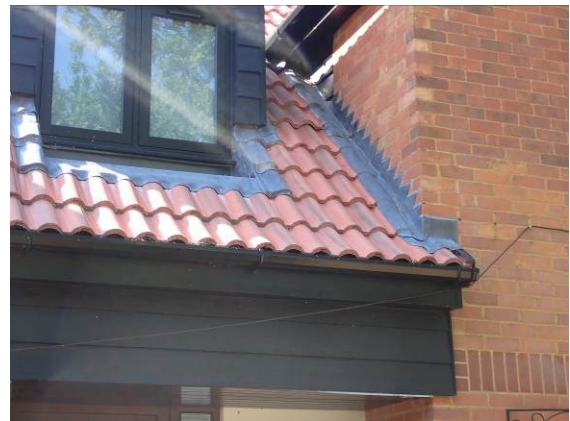
Photograph 2. The tightly fitted roof tiles and flashings.
