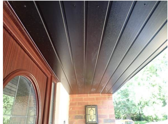
Photograph 4. Closely fitted fibre boards of existing unenclosed porch roof.
