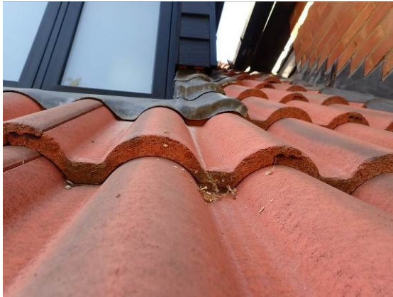
Photograph 3. Tightly fitted tiles of the roof above the porch.
