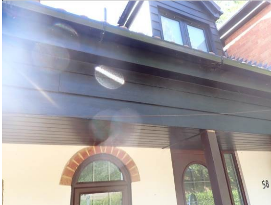
Photograph 5. The closely fitted fibre board fascias.
