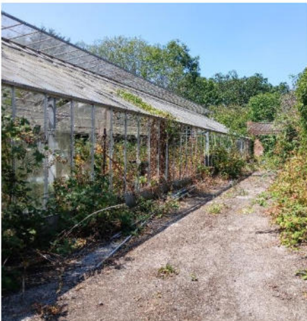
Disused greenhouses and hardstanding
