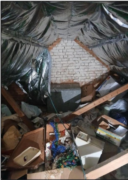
Loft space within building B9
