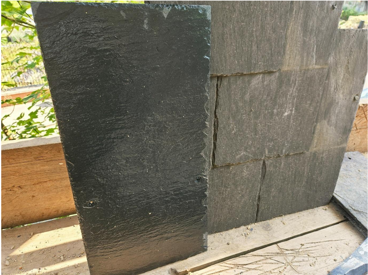
Photo 2: Photo of new slate (left side) against the old slate on the right.
