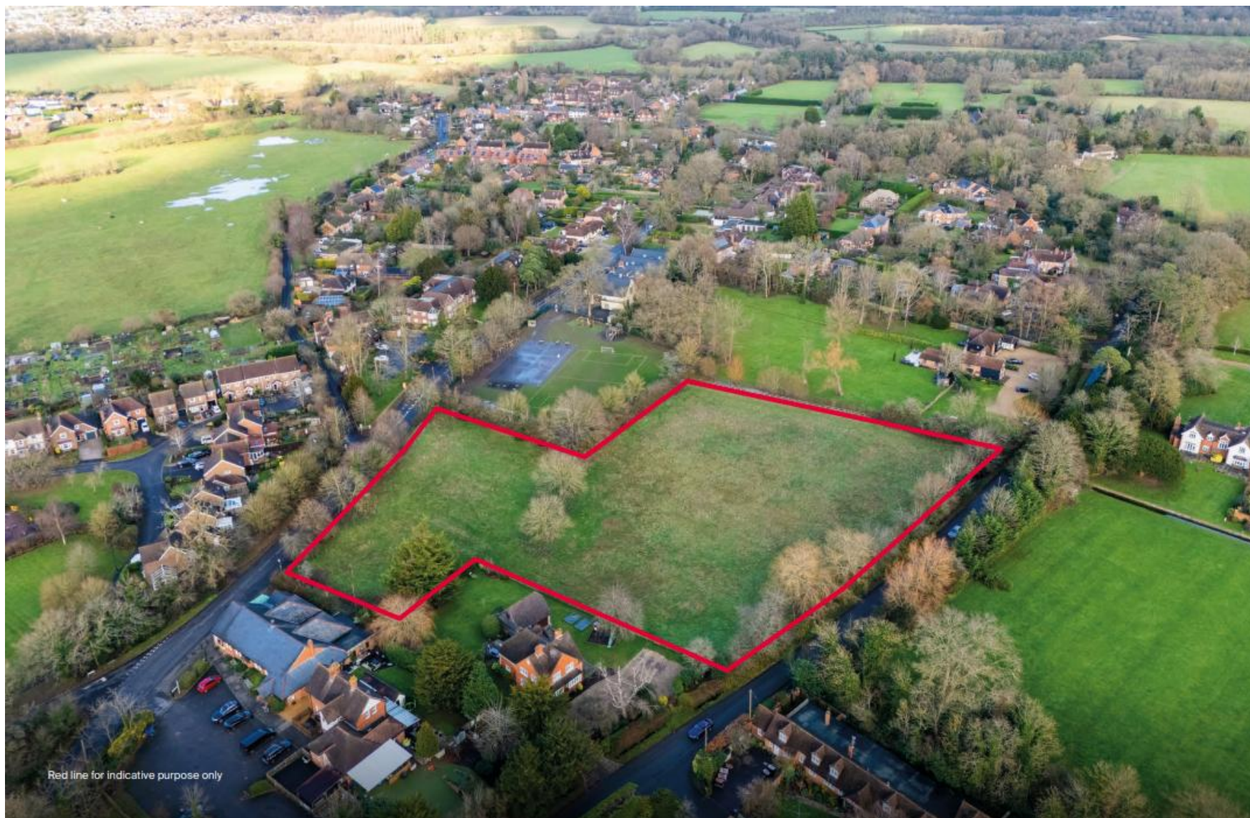
Fig. 1 Aerial view of the development area
