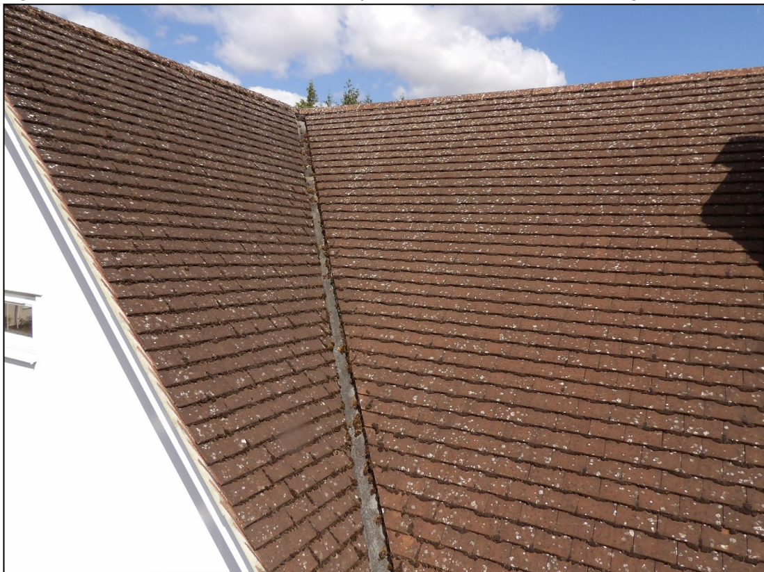
Figure 4. Example of roof tiles and valleys. 7 Buckhurst Grove, Wokingham. 08.07.25
