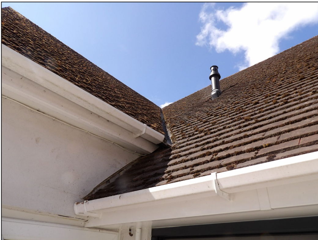
Figure 6. Example soffits/fascias. 7 Buckhurst Grove, Wokingham. 08.07.25
