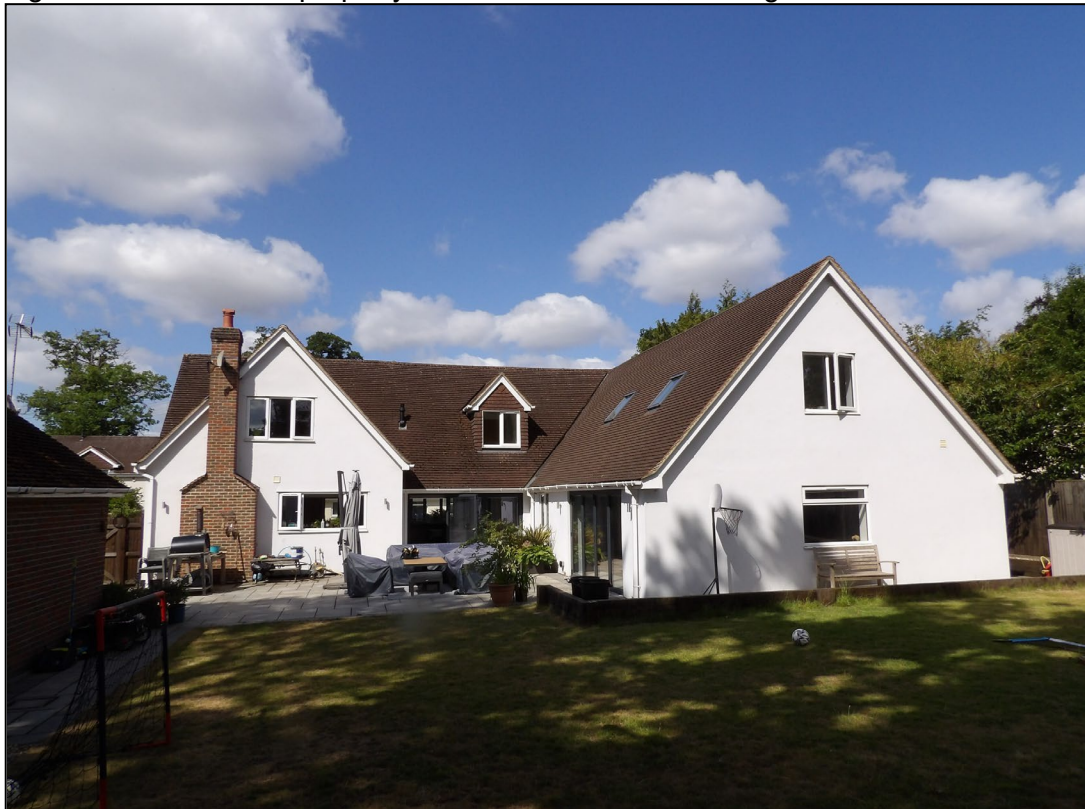
Figure 8. Rear view of property. 7 Buckhurst Grove, Wokingham. 08.07.25
