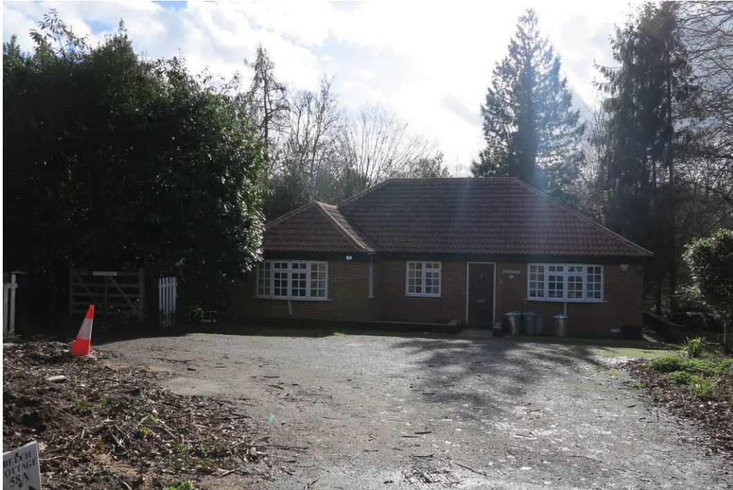
Plate 3. 58A Finchampstead Road was erected to the south-west of No.58 at the very end of the 20 th century
