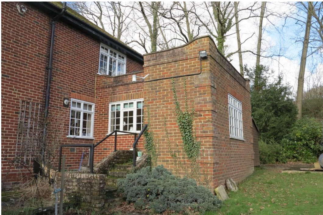
Plate 10. Kitchen/utility room extension (detail)
