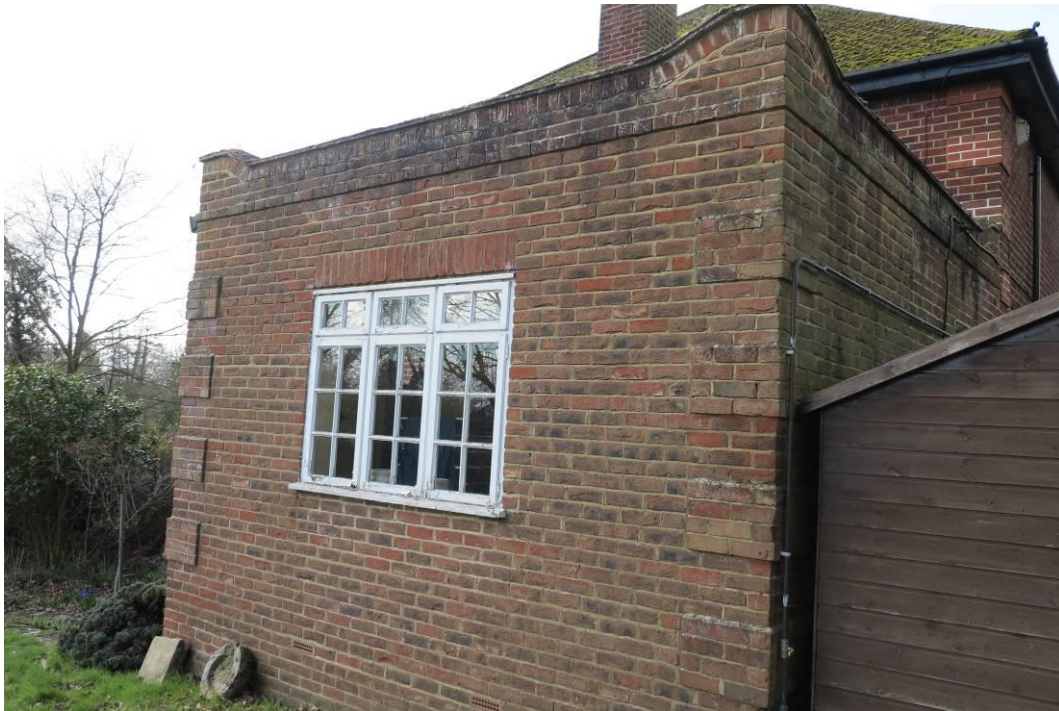
Plate 11. Kitchen/utility room extension (detail)
