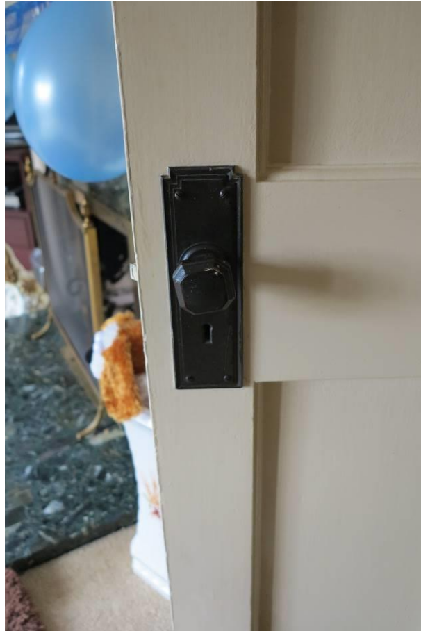
Plate 17. Detail of typical Bakelite door handles in the building
