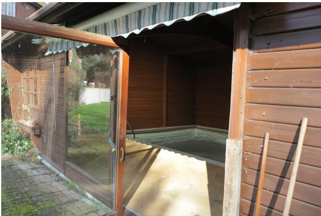
Plate 2. Free-standing swimming pool building in the rear garden
