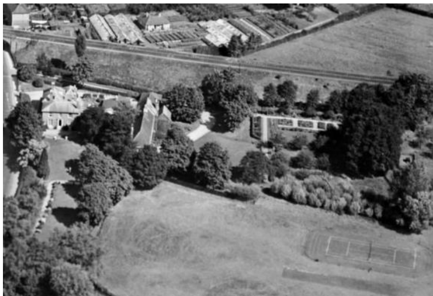
Fig.1. 1928 aerial image (HE ref. EPW023259) looking northwards. Southbrook is visible to the left and the application site just falls within the right-hand side of the image
