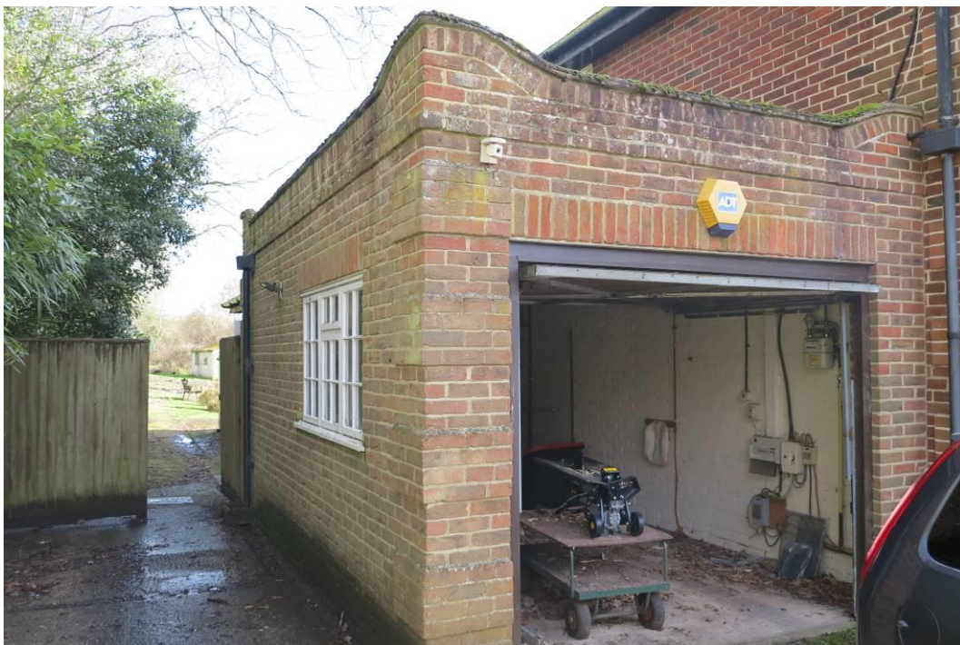
Plate 6. The garage on the northern side of the house
