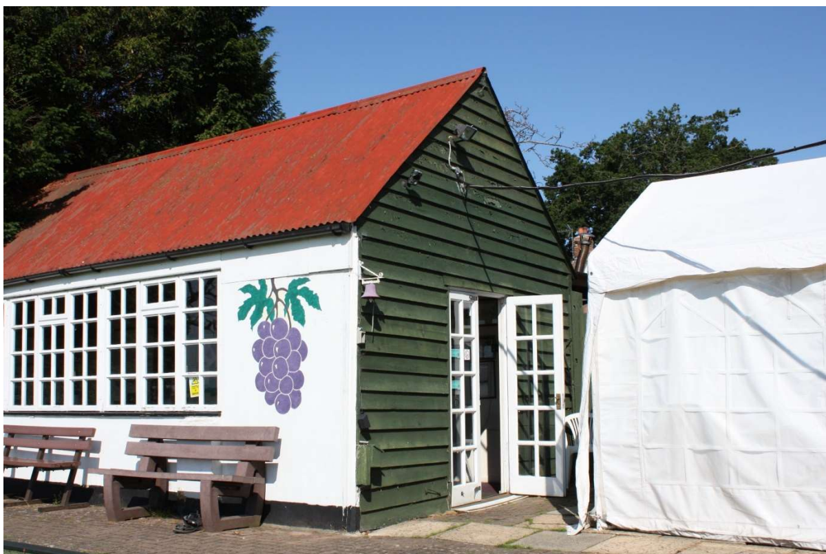
3. Main side, gable end with entry door. From East.
