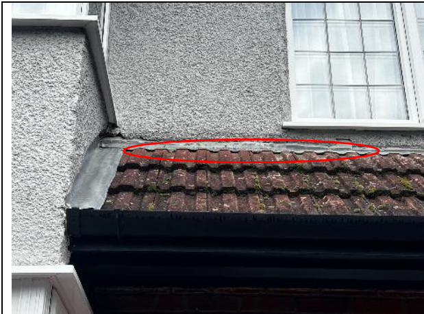
Figure 7: Lifted lead flashing on western entrance porch
