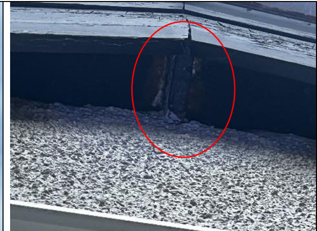
Figure 9: Gap at eaves on western gable apex
