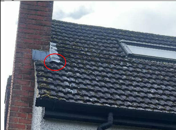
Figure 4: Lifted lead flashing on the east elevation
