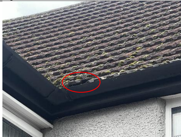
Figure 5: Lifted roof tile on the western elevation
