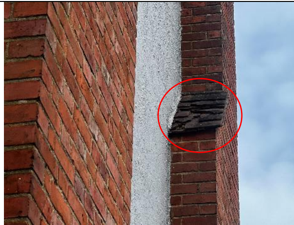
Figure 8: Slipped tiles on southern elevation
