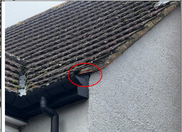
Figure 6: Gap in south-western soffit
