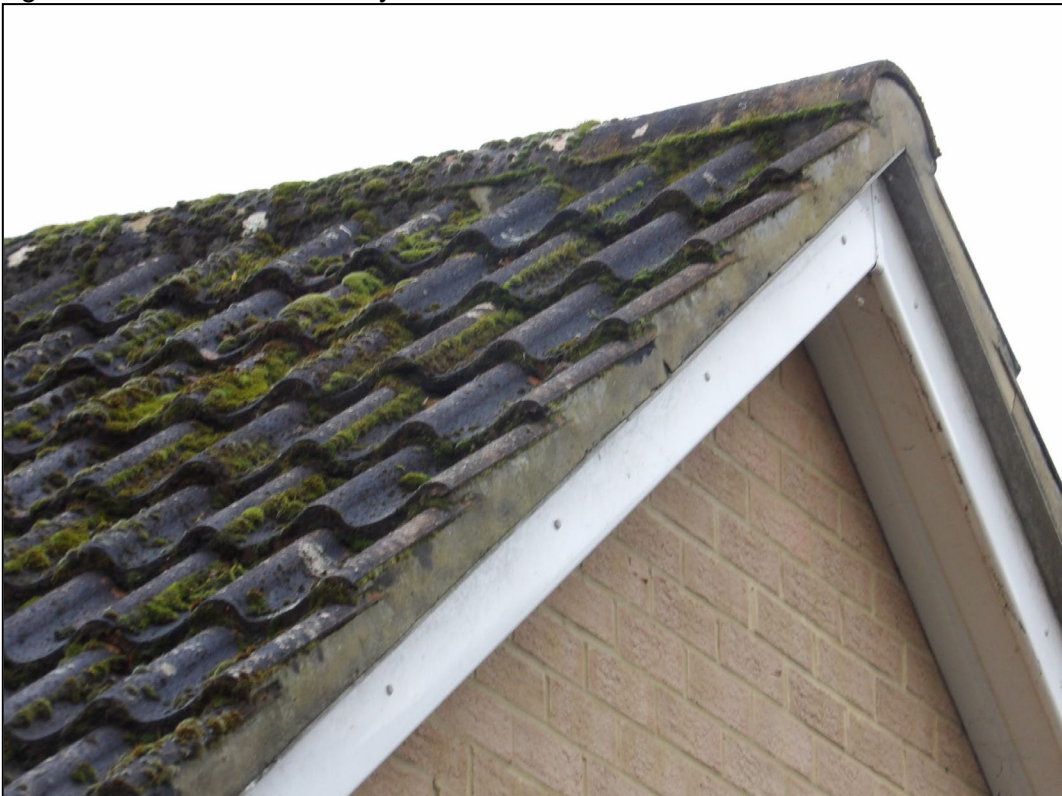
Figure 10. Example sealed verge and uPVC soffits and fascias on garage. 65 Egremont Drive, Lower Earley. 09.12.25
