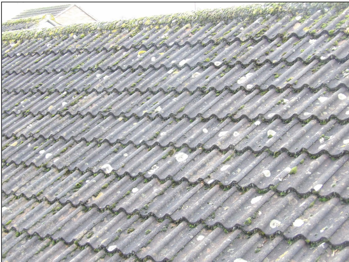
Figure 4. Example of interlocking roof tiles. 65 Egremont Drive, Lower Earley. 09.12.25
