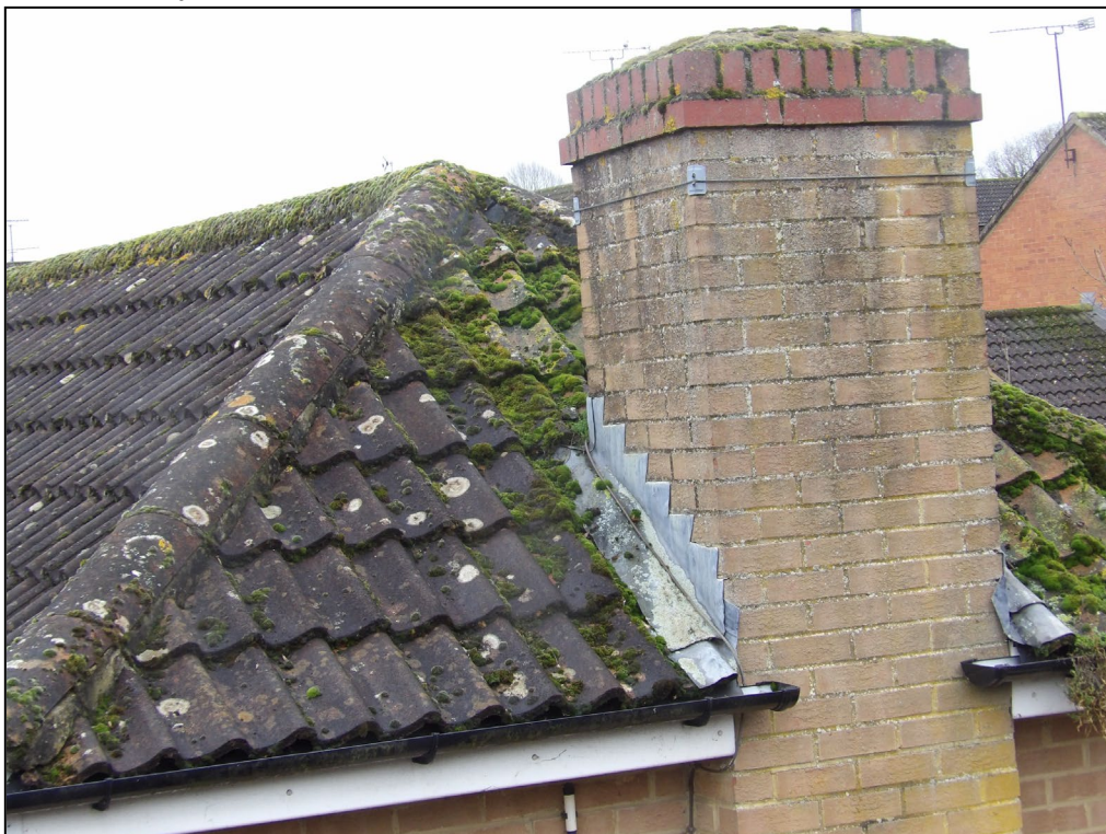
Figure 6. Example sealed lead flashing around chimney stack. 65 Egremont Drive, Lower Earley. 09.12.25
