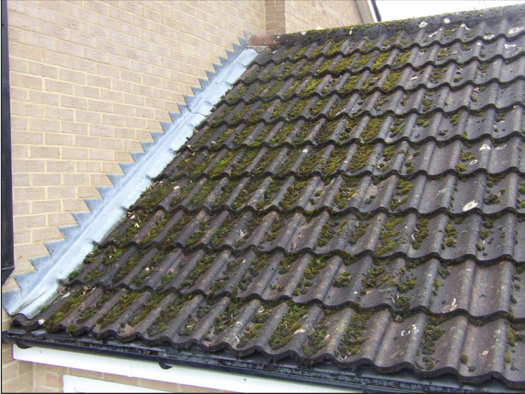
Figure 9. Example sealed roof and ridge tiles on garage. 65 Egremont Drive, Lower Earley. 09.12.25
