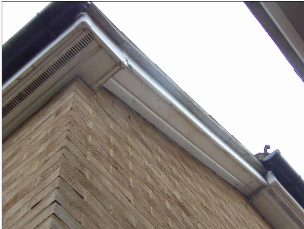
Figure 8. Example sealed uPVC soffits and fascias. 65 Egremont Drive, Lower Earley. 09.12.25
