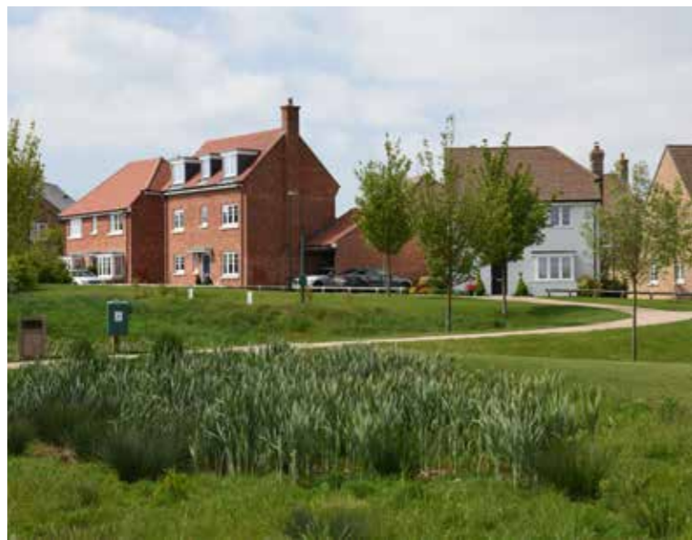
Houses fronting onto a landscaped attenuation basin
