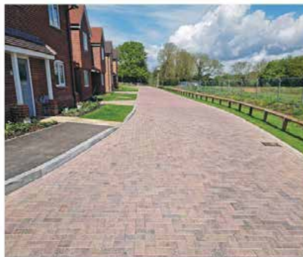
Block paving to roads/shared surfaces
