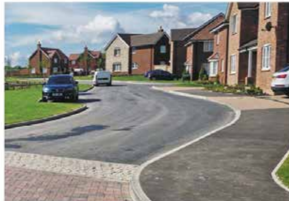
Bitumen macadam to road and pavements
